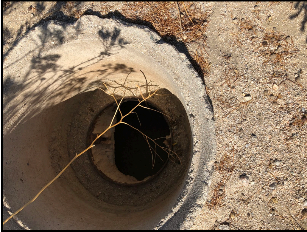
Exposed concrete irrigation structures leading to below ground lines.
