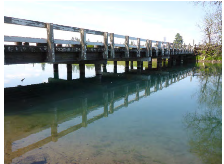
Photo 4.4-3. View of existing bridge, facing northwest.
