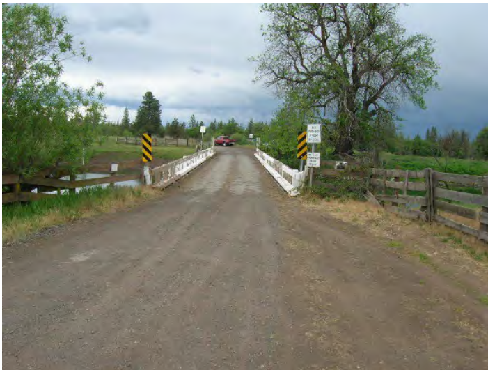
Photo 4.4-2. View of existing bridge, facing north-northwest.
