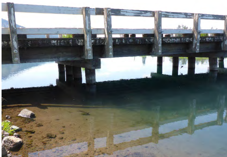
Photo 4.4-5. Existing bridge railing.
