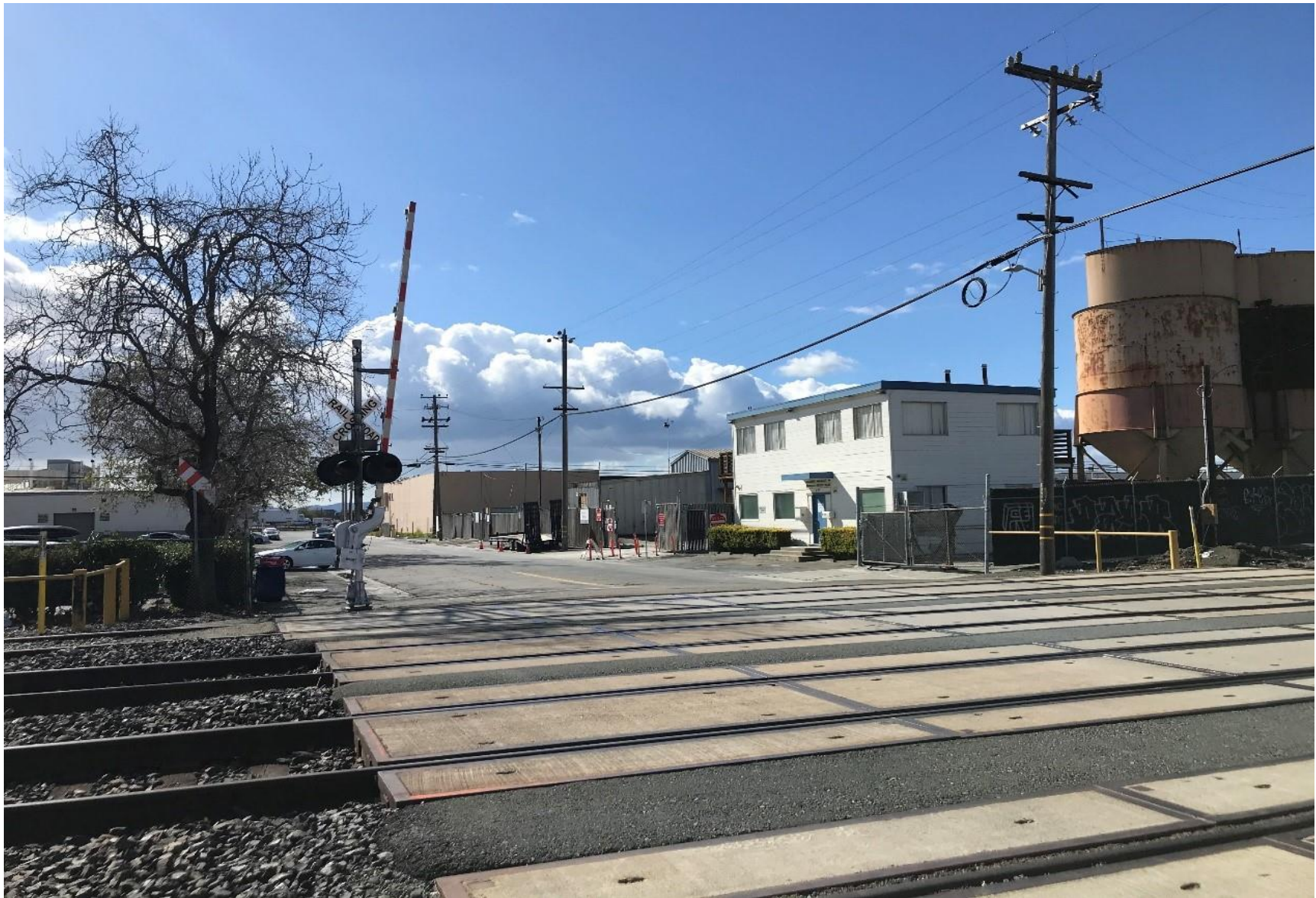
Figure 2 Virginia Street Crossing - Existing Conditions
