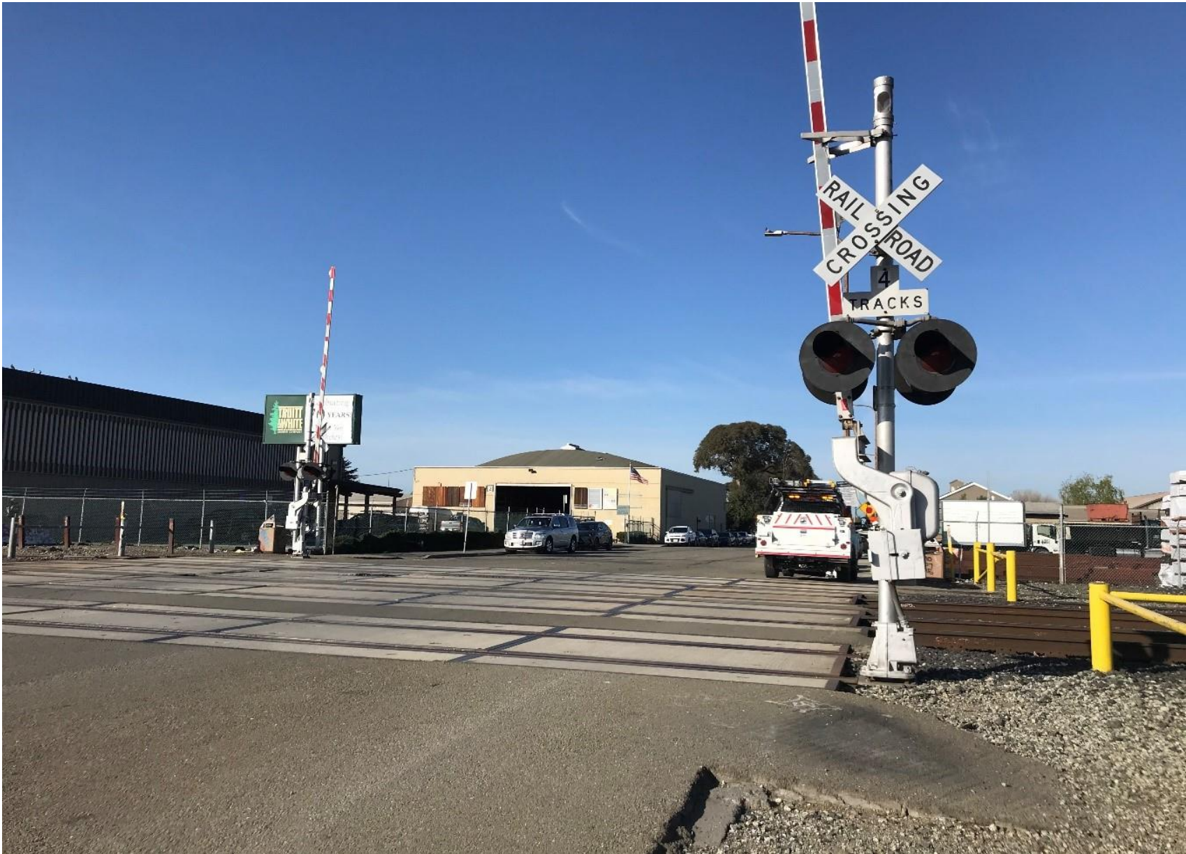
Figure 3 Hearst Avenue Crossing - Existing Conditions
