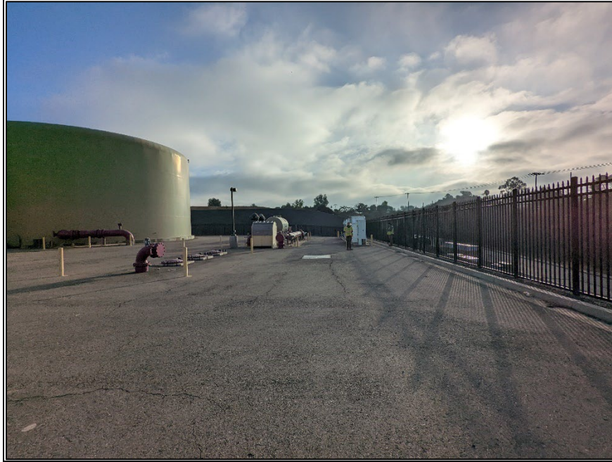
Photo 3. Representative photo of existing facilities adjacent to the B10.3.3 booster site.
