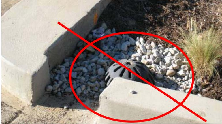
**Figure 6: Incorrect Placement of an Overflow Inlet.**
