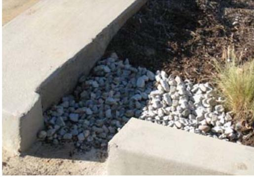
**Figure 2: Curb Cut located in a Bioretention Facility**
