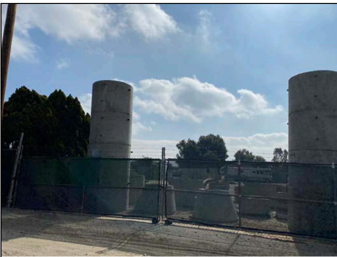
11. View of the southwest adjoining property
