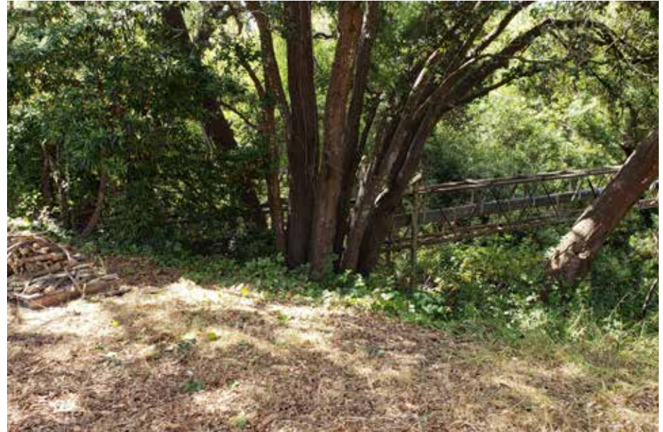
Photo 10. Pipeline elevated crossing, coast live oak proposed for removal in foreground (Manhole 48).
