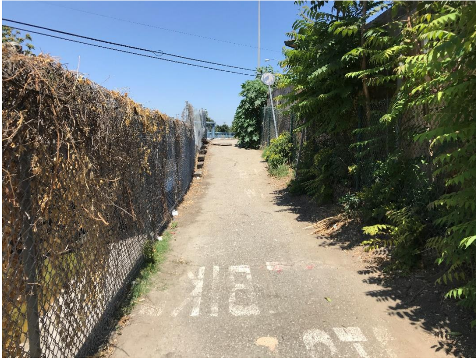
Facing northwest toward bike lane that runs adjacent to Compton Creek.
