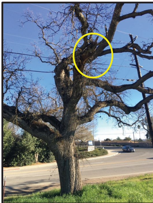
Photo 3 - View of broken branch west side of tree circled in yellow.
