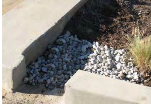
Figure 2: Curb Cut located in a Bioretention Facility
