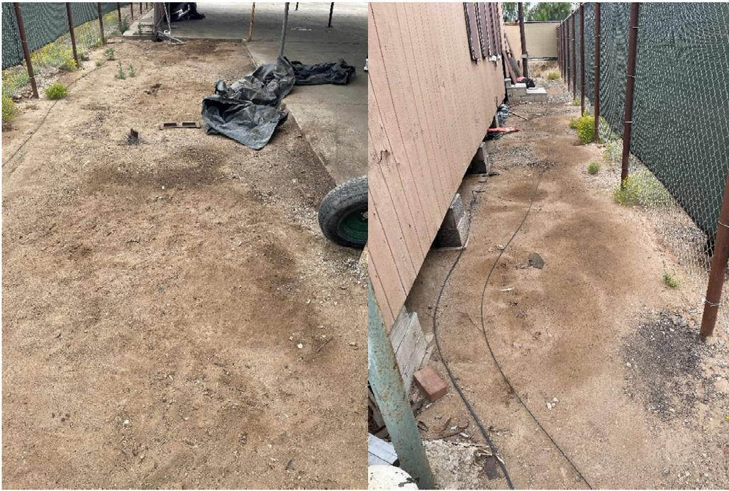
Photo 5: View of surficial soil staining near the former fleet maintenance area on the western portion of the site.
