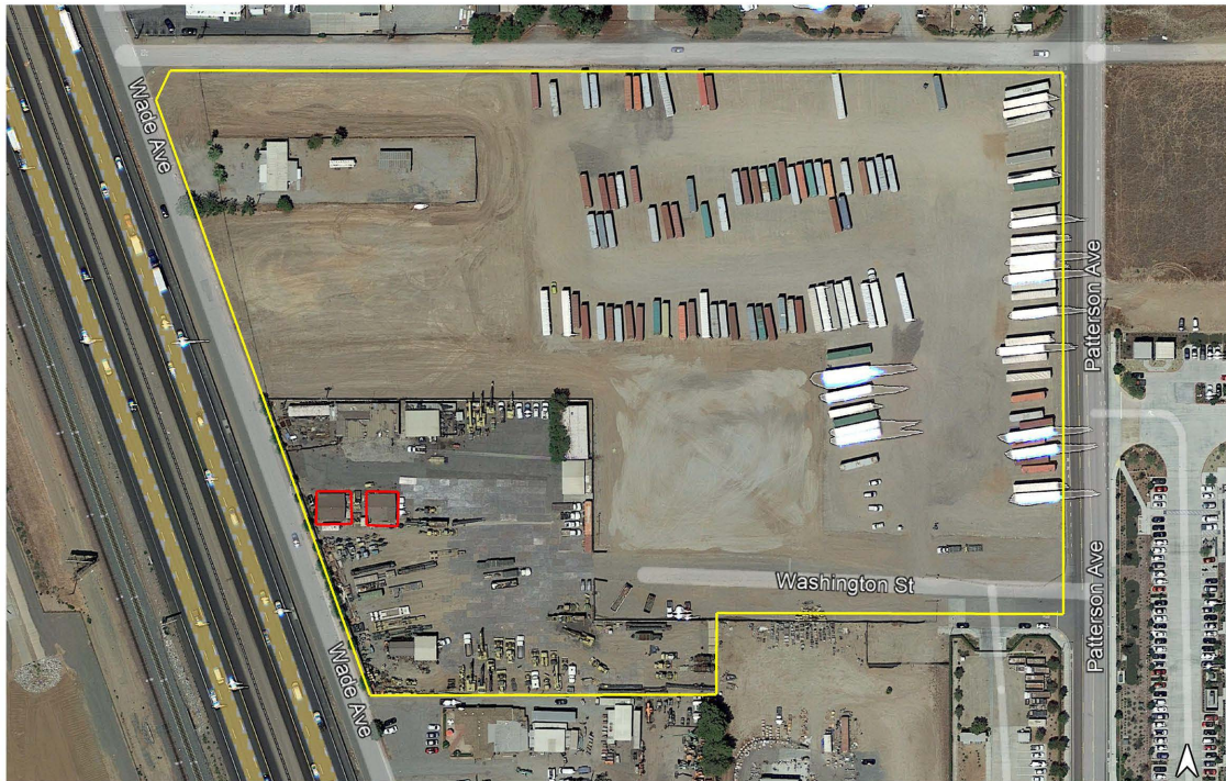
Plate 3.2–3: Aerial overview of the project (yellow) showing the buildings recorded as Temp-1 (red). (Image courtesy of Google Maps)
