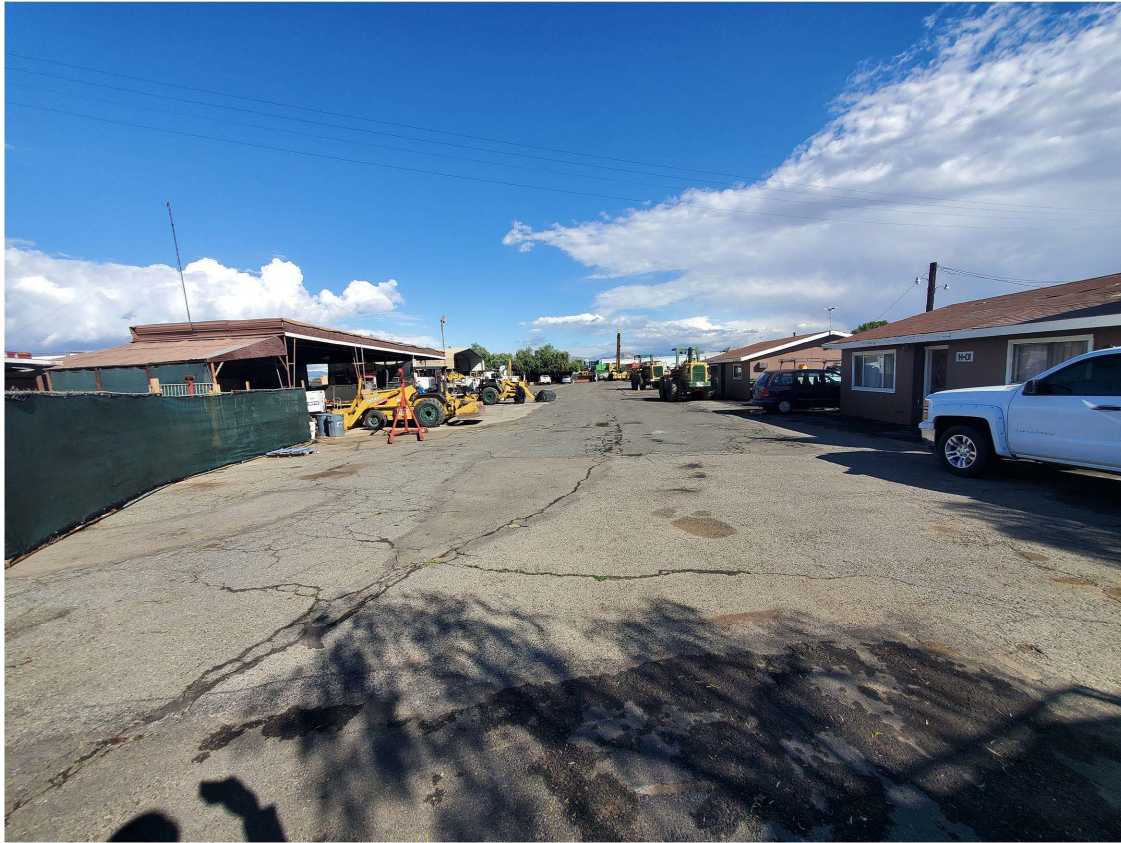
Plate 3.3–8: Concrete asphalt pavement surrounding the residences, facing east.
