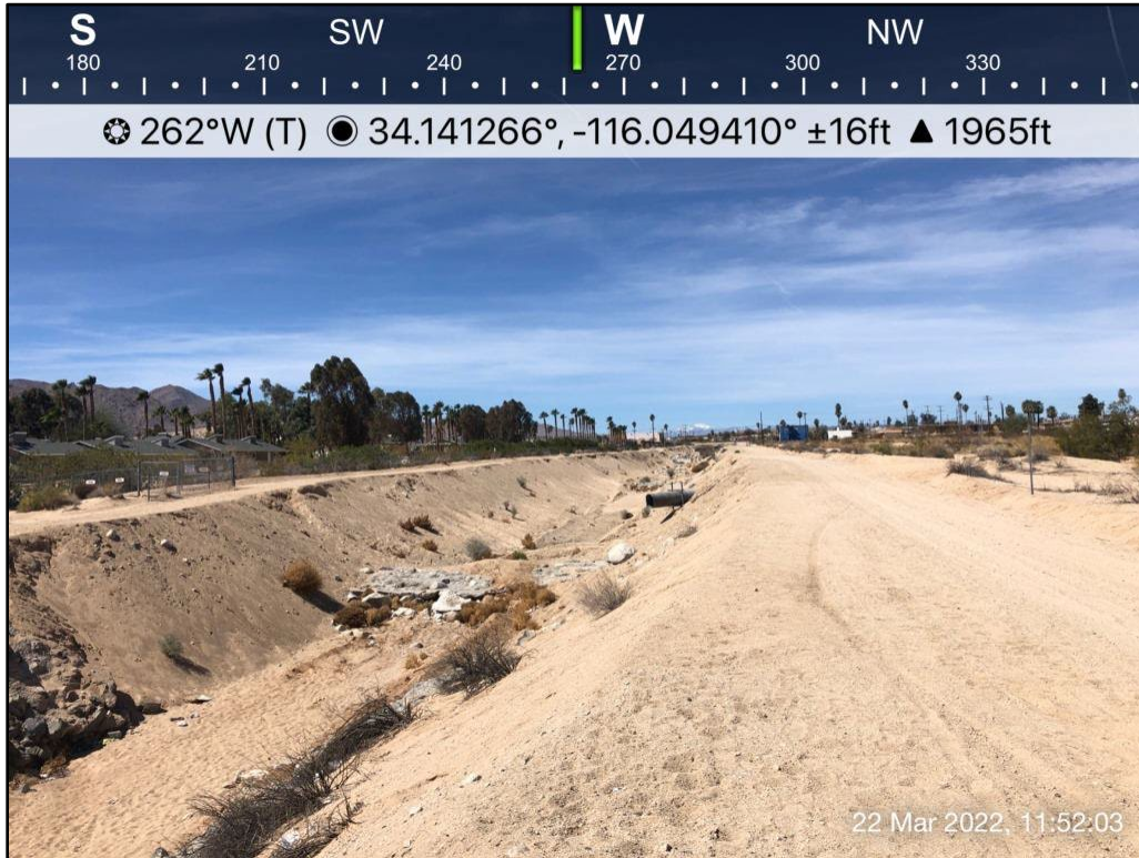
Photo 3. Examples of potential burrowing owl habitat (riprap, concrete slab with cavities beneath).
