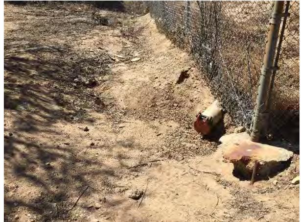
**Photo 6:** Pipe that releases water periodically into drainage within the center of the project site. Facing southwest.
