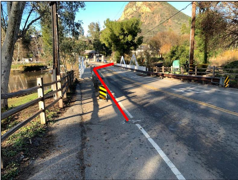
c. Proposed sewer bypass pipe alignment on bridge and shoulder
