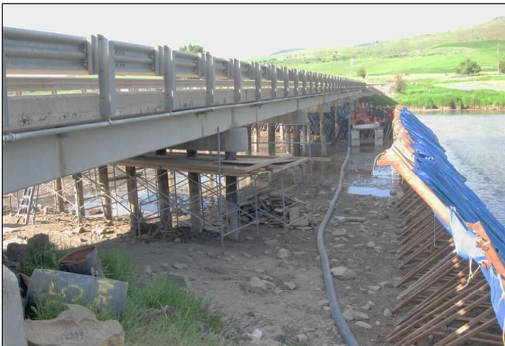
b. Example installed cofferdam system
