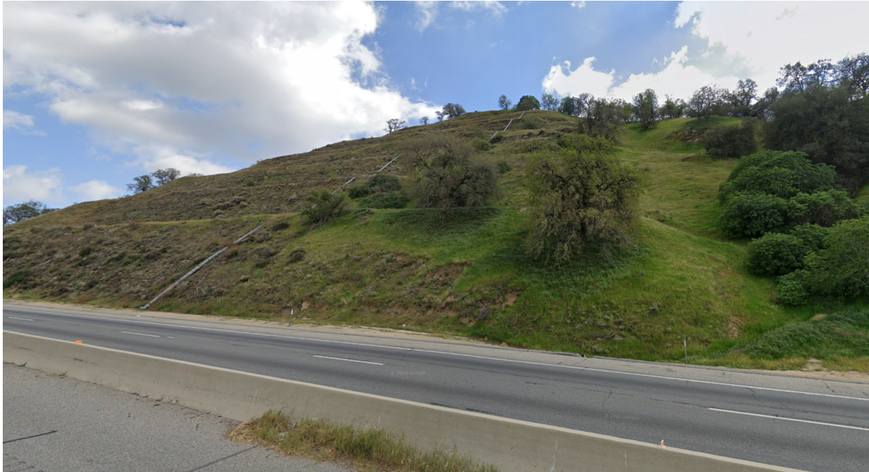
Figure 8 - Photo of multi-tiered benched cut slope at post mile 77.66
