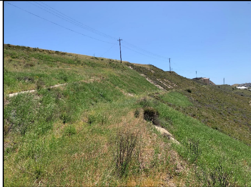
b. Southern portion of the capacity increase area, facing southeast (4/19/22)
