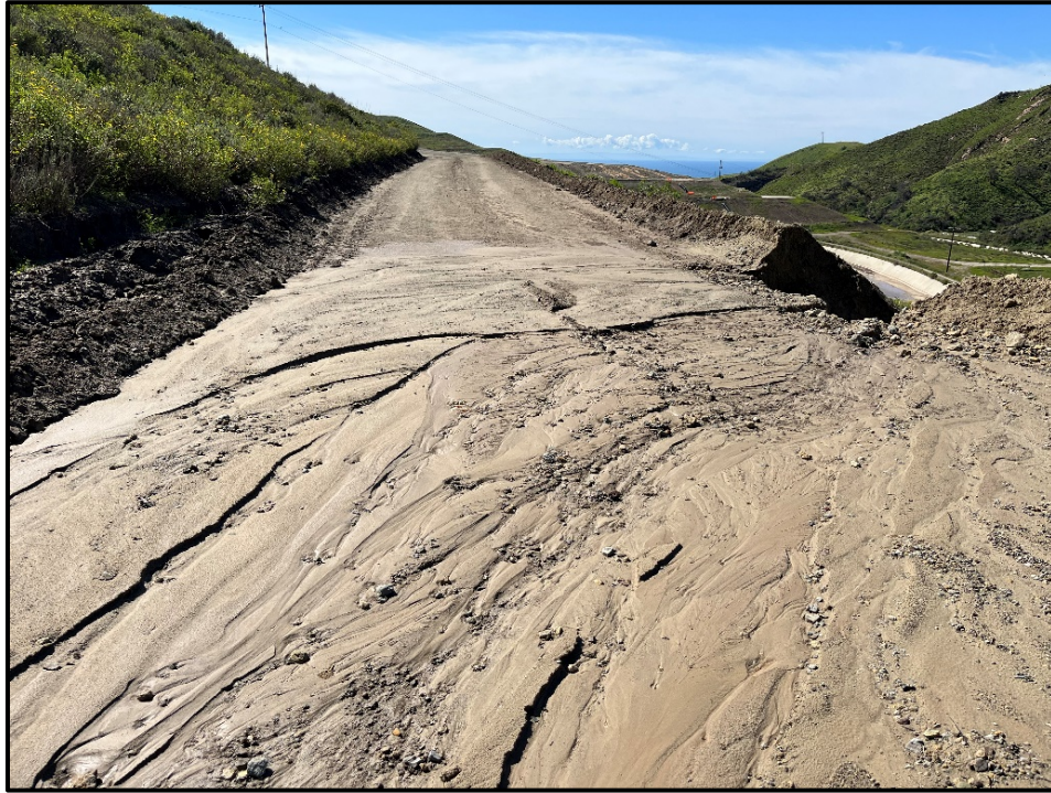
Figure 3. Overview of sheet washing at access road along southern edge of Survey Area, facing east
