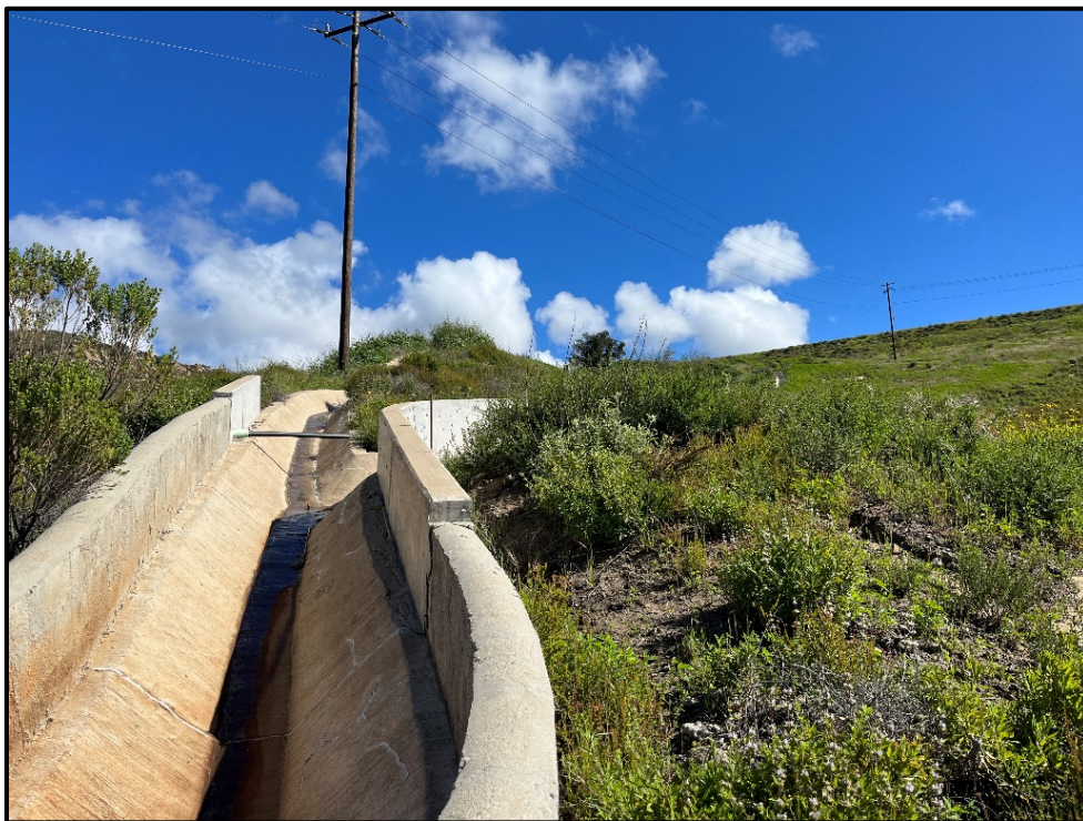
Figure 4. Overview of V-ditch alignment, facing northeast
