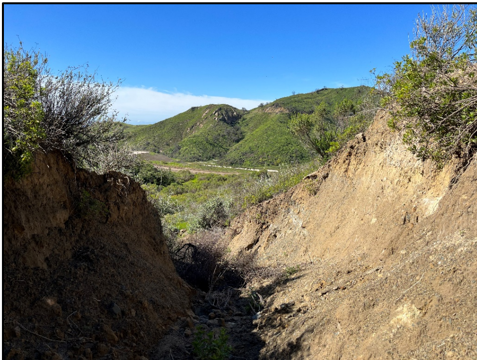
Figure 2. Overview of gully, facing southwest
