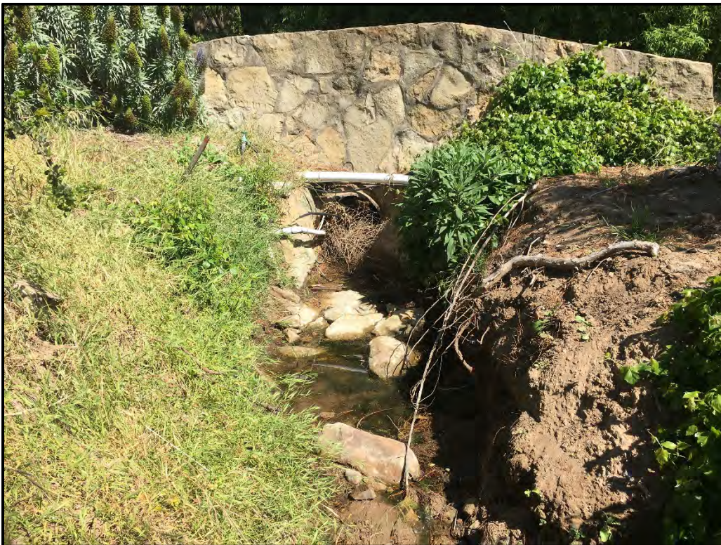
Photo 2: Existing 24 inch culvert under the bridge (Aspect: North). Photo taken 05/08/2020.
