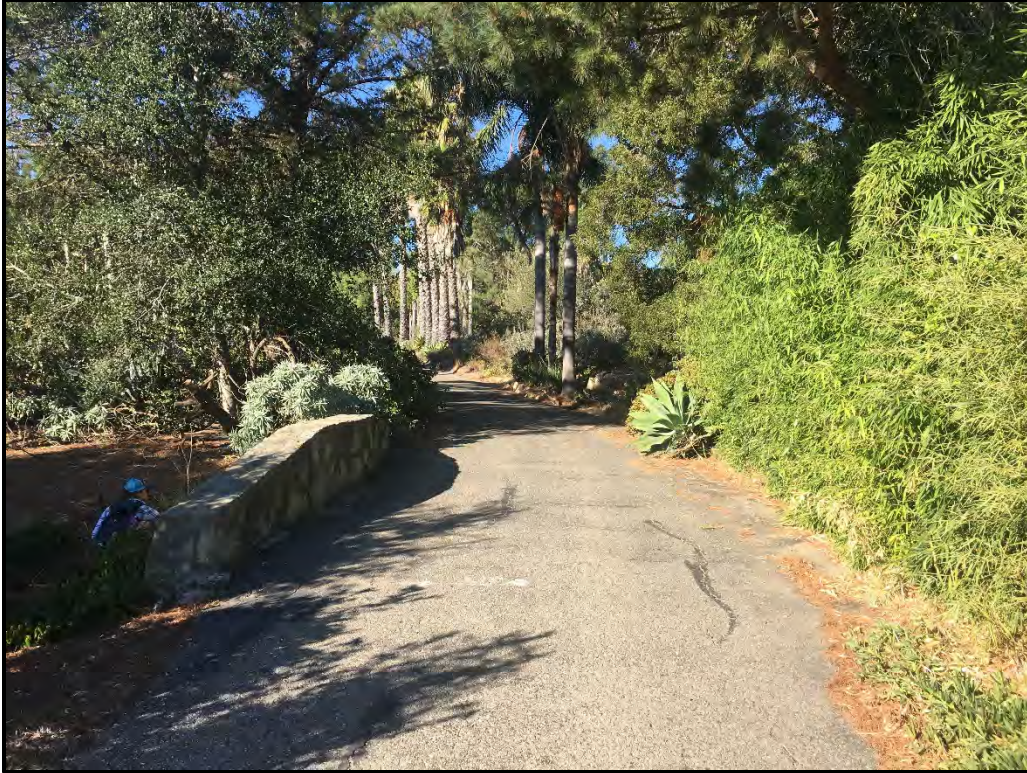
Photo 1: Main access driveway and existing bridge (Aspect: West). Photo taken 10/31/2019.
