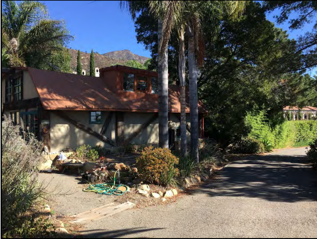
Photo 15: Existing cottage adjacent to the ephemeral drainage and bridge (Aspect: East). Photo taken 10/31/2019.
