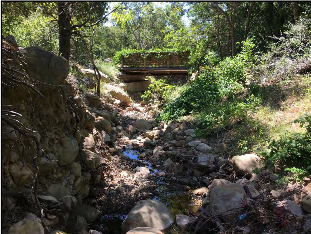
Photo 6: Lower portion of Oak Creek and the bridge along the private road southwest of the Project Area. (Aspect: South). Photo taken 05/08/2020.
