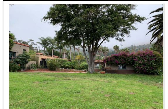
Photograph 1. The proposed Project would result in creation of four residentially developable parcels. Construction activities associated with the Vesting Tentative Tract Map would include demolition of the existing structures and hardscapes, limited grading, and construction of utilities and drainage improvements as well as a new shared-access driveway.
