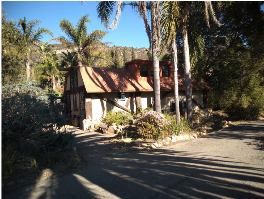
Figure 34, South elevation of Garage #2, looking northeast
