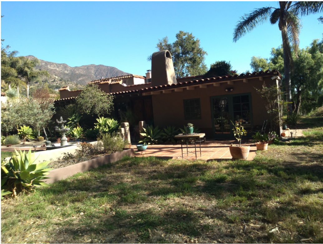
Figure 19, West Elevation looking east
