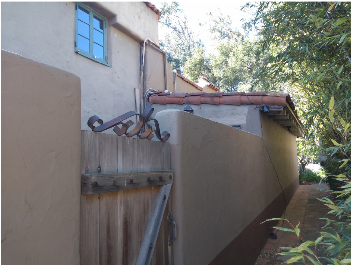
Figure 23, North elevation of house, looking west
