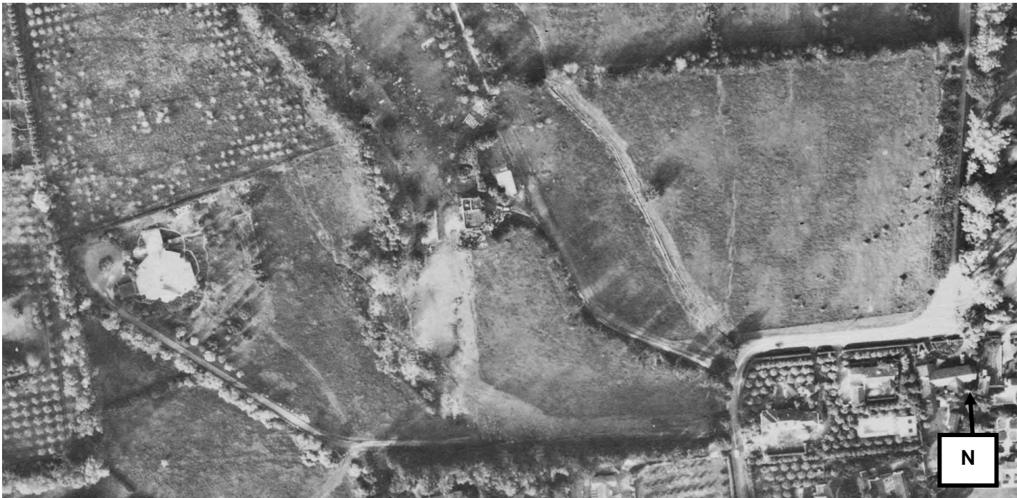
Figure 12, 1969 Aerial Photograph (Map and Imagery Collection, Special Collection, Davidson Library, University of California, Santa Barbara, Flight hb-nn_178, begun January 26, 1969) (depicting deterioration of buildings and landscaping)
