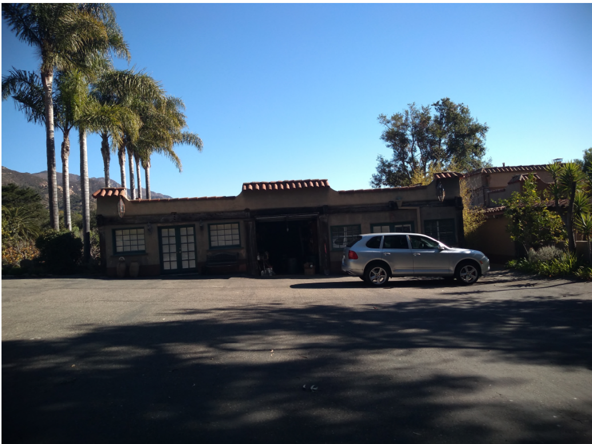
Figure 31, West elevation of garage/studio, looking east
