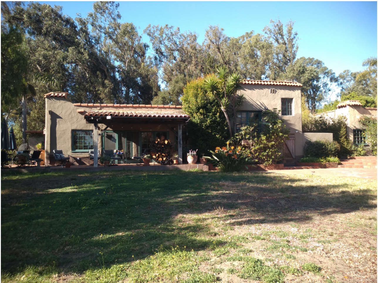
Figure 26, East elevation of house, looking west
