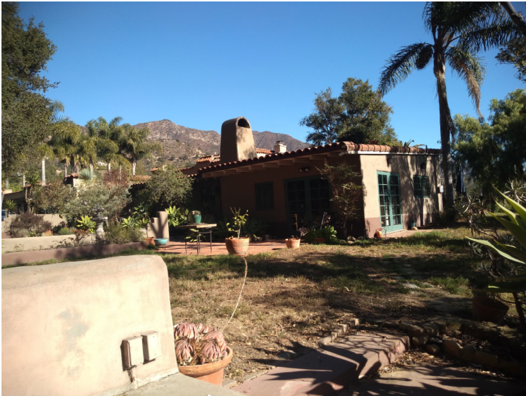
Figure 22, Southwest corner of the house looking northeast
