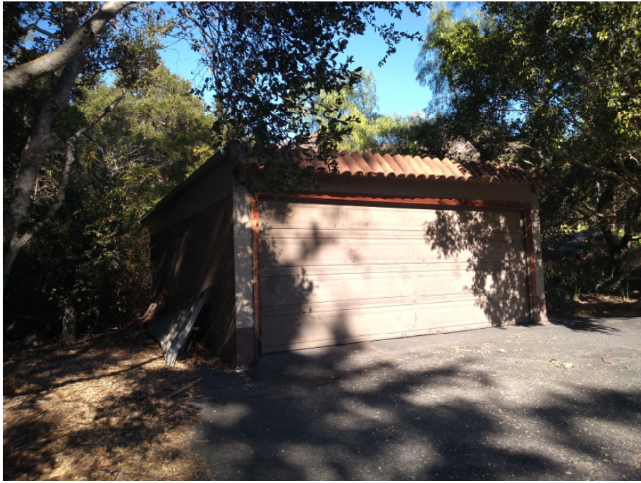
Figure 33, South elevation of Garage #2, looking northeast
