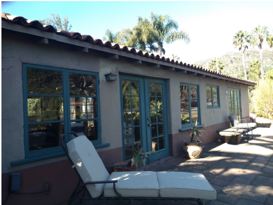
Figure 27, East elevation of the guesthouse, looking north
