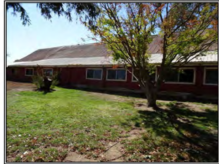
Looking southwest at Structure C.
