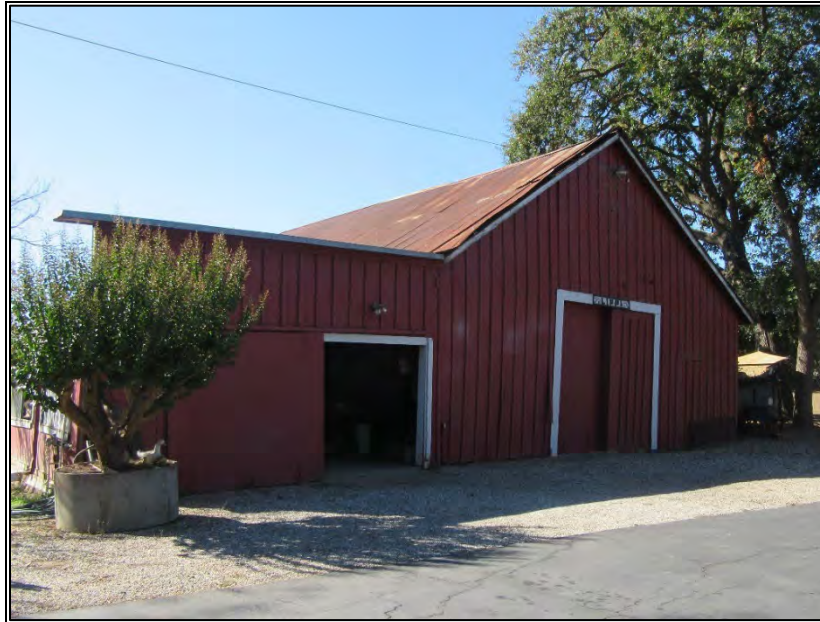
Figure 7. LR-02 (view south; September 29, 2022).
