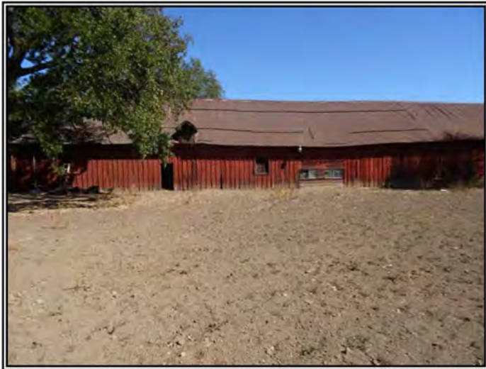
Looking east at Structure C.
