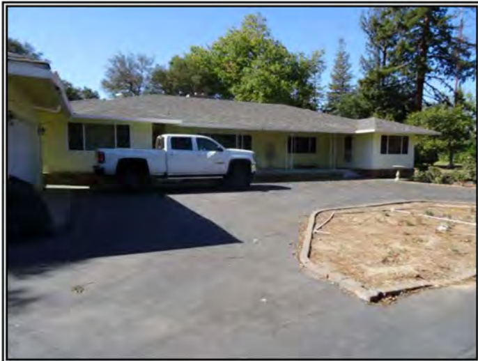
Looking northwest at Structure E.
