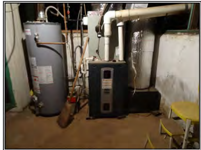
Looking at the basement of Structure B.
