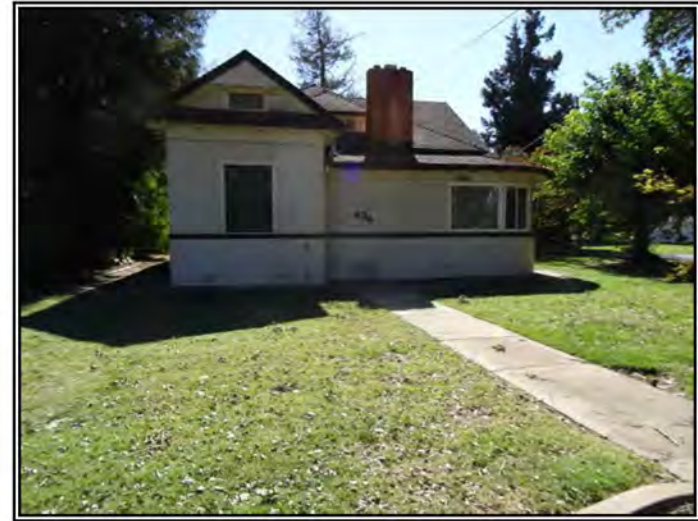
Looking south at Structure B.
