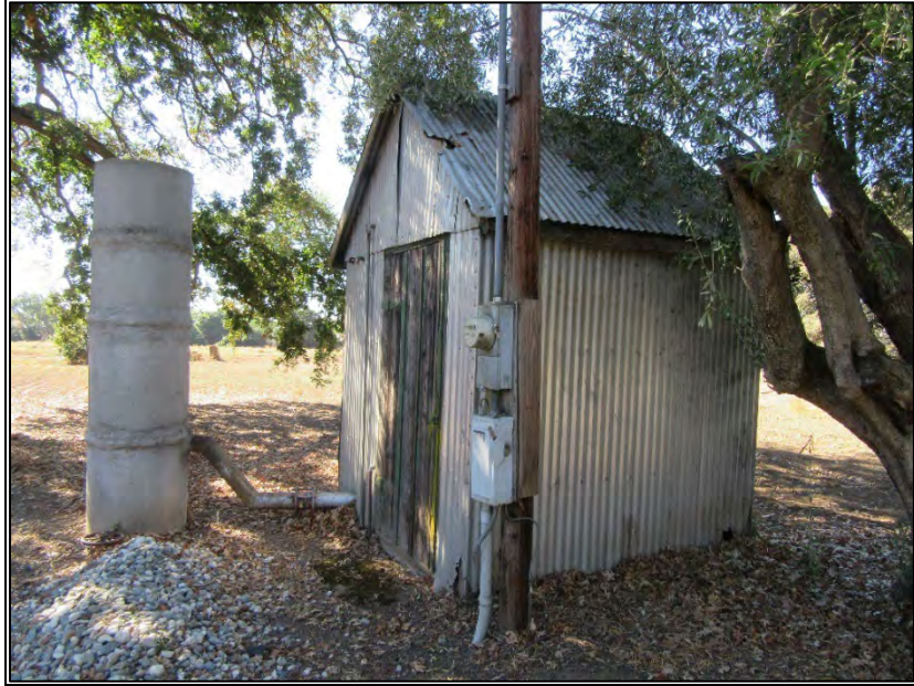
Figure 8. LR-03 (view south; September 29, 2022).
