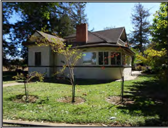
Looking southeast at Structure B.
