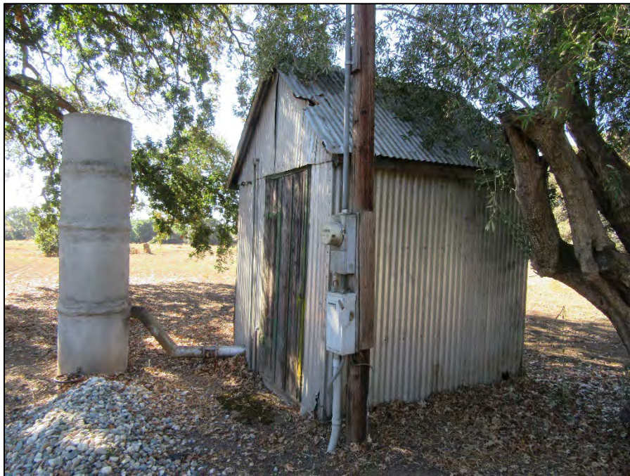
Figure 5. LR-03 (view south; September 29, 2022)
