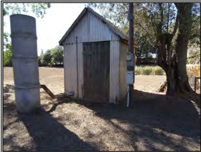
Looking southwest at the pump house and concrete irrigation standpipe .
