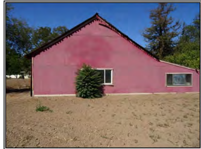
Looking north at Structure C.
