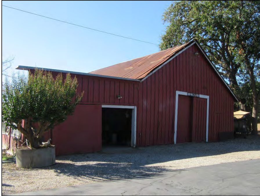
Figure 4. LR-02 (view south; September 29, 2022)
