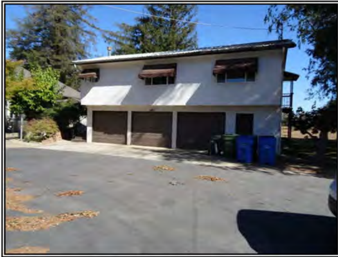
Looking northeast at Structure G.
