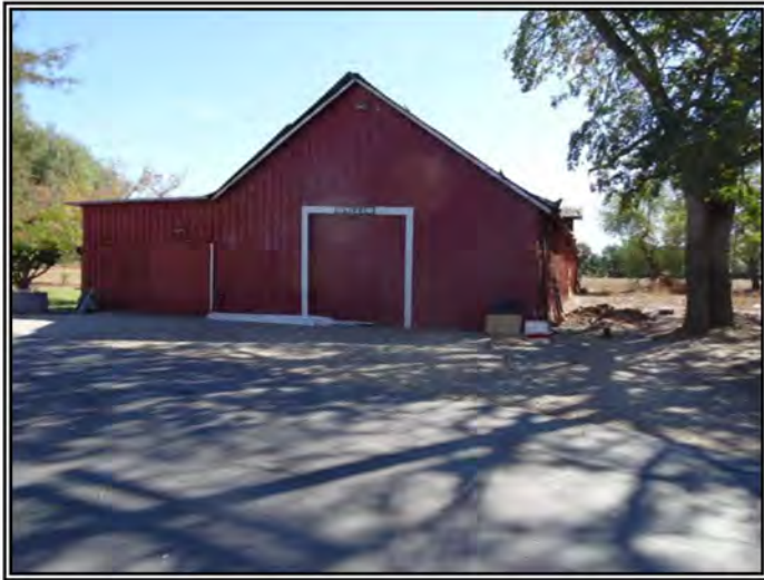
Looking southeast at Structure C.
