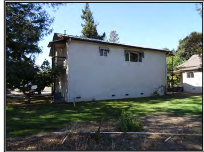
Looking northwest at Structure G.
