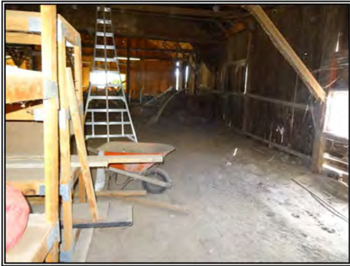
Looking at the interior of Structure C.
