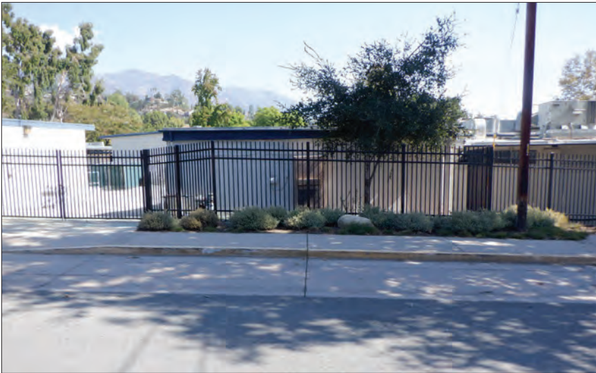
View from Gould Avenue at the western campus boundary showing the view of the existing portable structures (proposed to be removed and replaced with a building), facing east.
