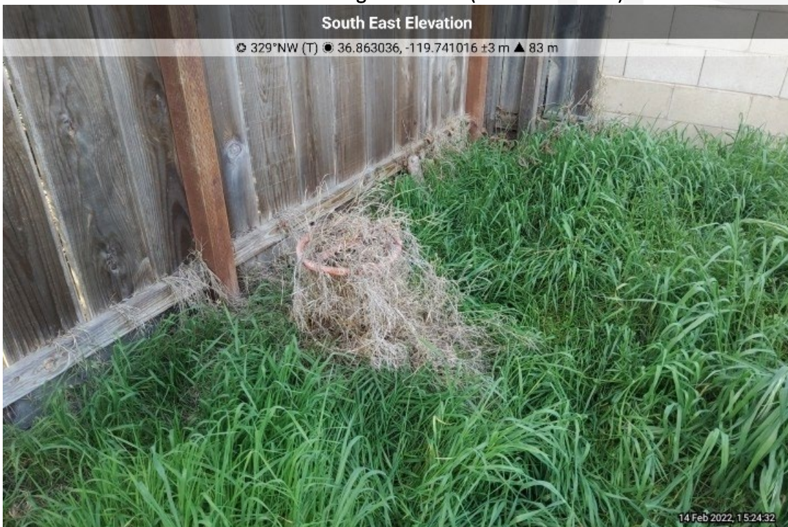
Photo 10 – Water Irrigation Valve (View Northwest)
