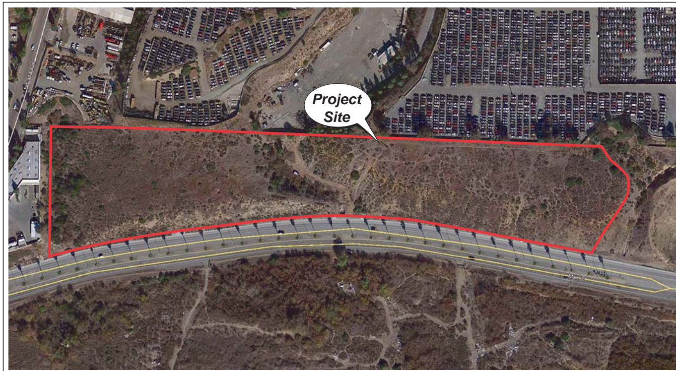
Reference: Google Earth Aerial Photograph Chula Vista, California - December 2020
