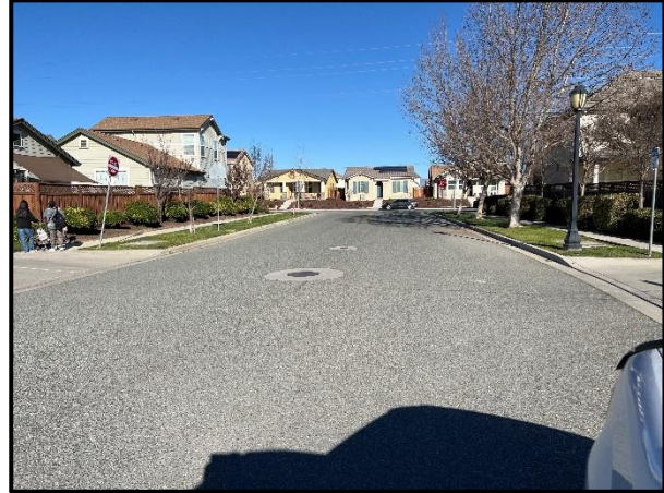
Photo 20. Location of proposed 6-inch pipeline section along Calcagno Street. Residential zone, view east. January 26, 2023.
