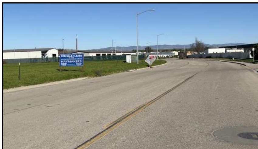
Photo 2. View of proposed pipeline location within road in northeast portion of the Study Area, facing east. January 26, 2023.
