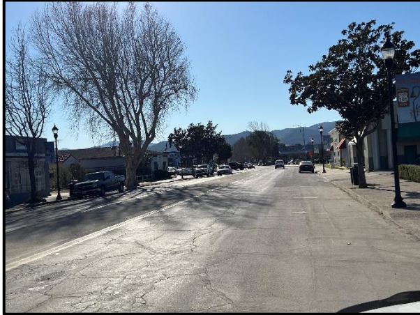
Photo 19. Location of proposed 8-inch pipeline section along Broadway Street. Commercial zone, view southwest. January 26, 2023.
