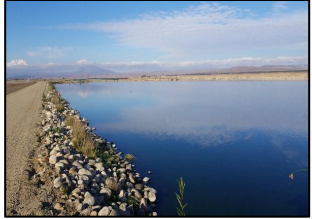
Photo 14. Active treatment pond, view north. December 7, 2021.
