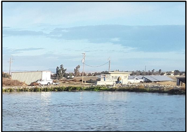
Photo 16. Associated WWTP facilities including office, storage container, and parking, view east. December 7, 2021.
