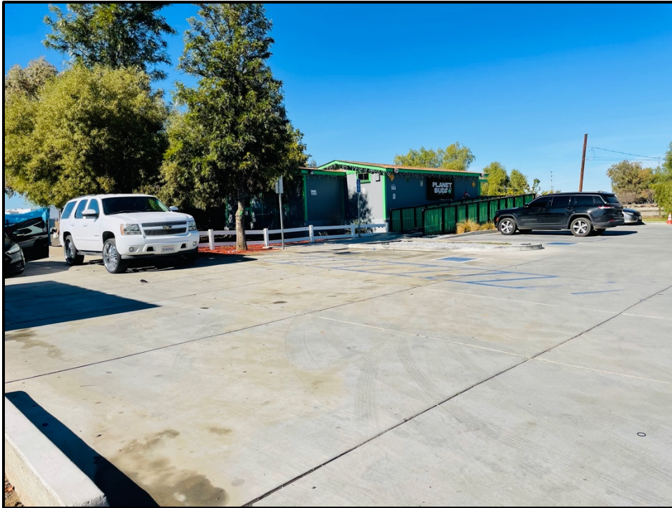
Plate 1: Overview of the apothecary store and paved areas within APN 300-210-014 (3060 Wilson Avenue), facing northwest.
