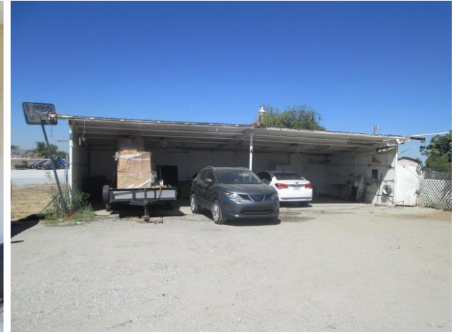
9. Carport/storage at 3040 Wilson Avenue.
