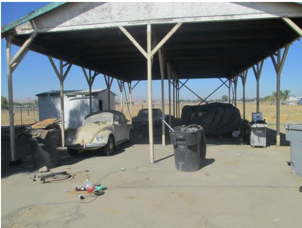
4. Carport/canopy at 2980 Wilson Avenue.
