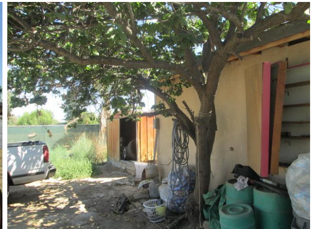
12. Rear of residence (foreground) and storage shed (background) at 3040 Wilson Avenue.
