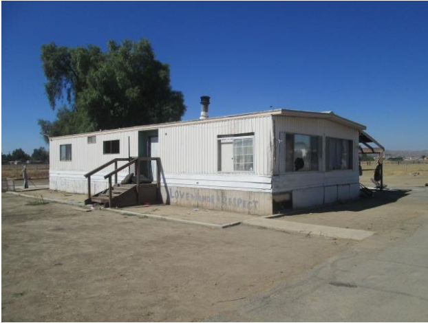
1. Residence at 2980 Wilson Avenue.
