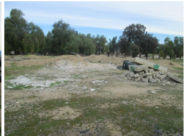
30. Debris and soil piles at 3060 Wilson Avenue.
