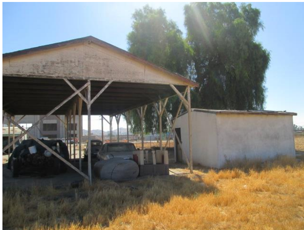
5. Carport/canopy and shed at 2980 Wilson Avenue.
