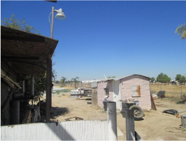
13. Carport/storage building (left) and dwelling unit (right) at 3040 Wilson Avenue.
