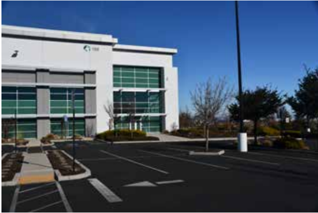
Enhanced Building Entries
