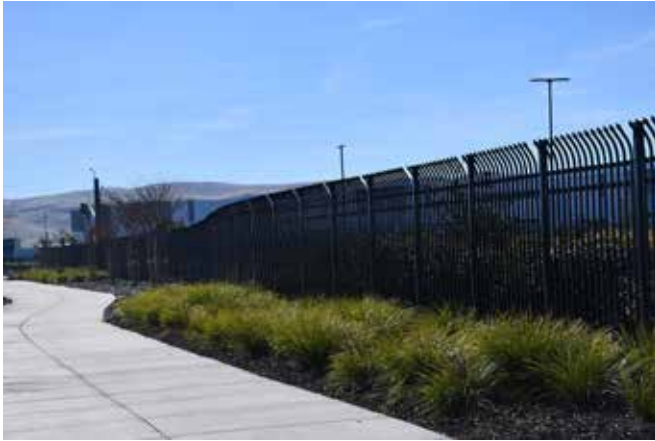
Typical Tubular Steel Fencing
