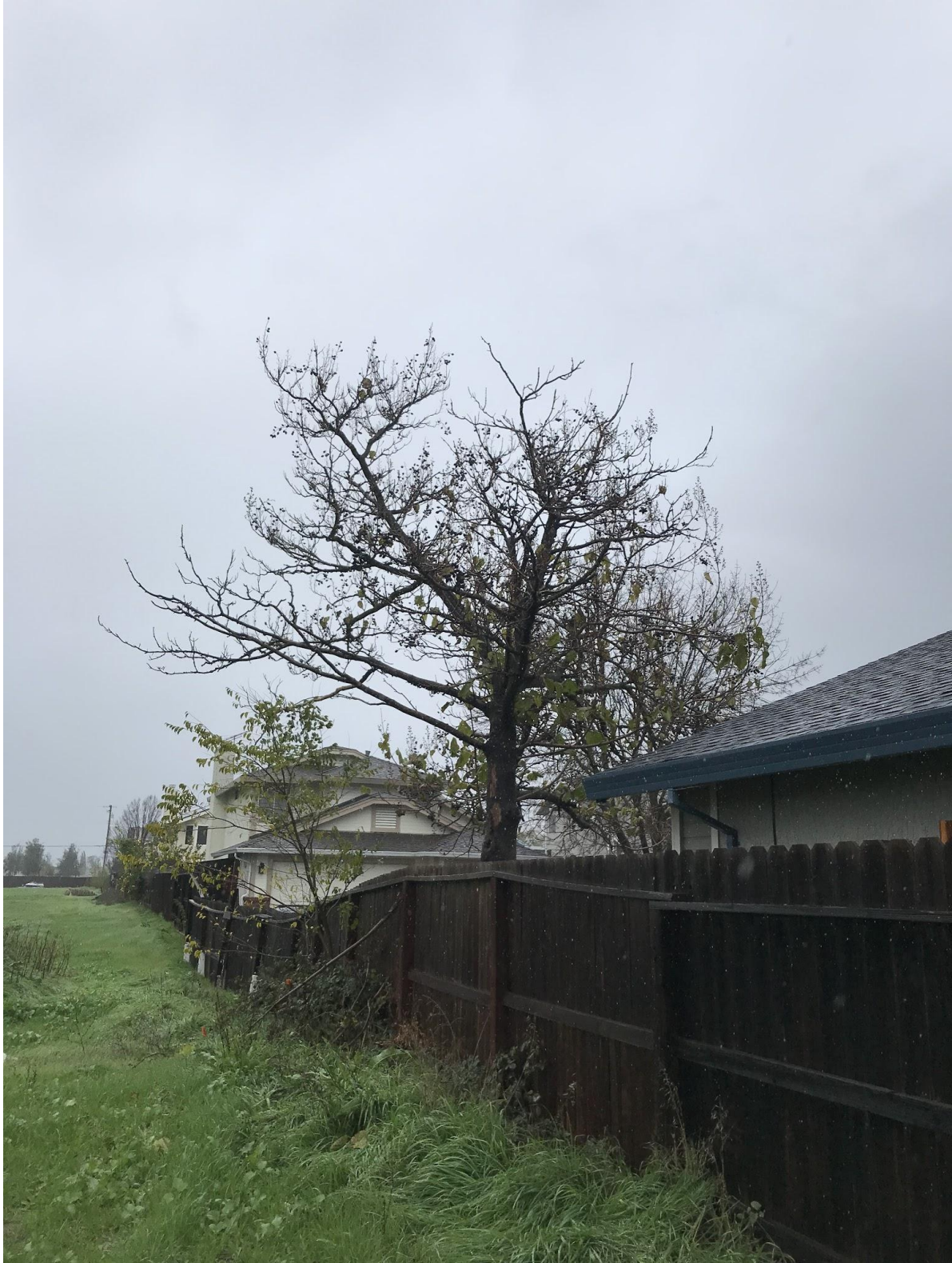
Photo 3. Tree #3 at 8180 Cliffe Way is in poor condition with large deadwood over the parcel; remove deadwood over the parcel and install tree protection fencing along the CRZ to the existing fence.
