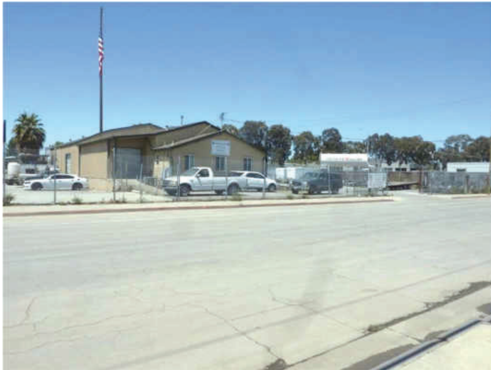
E-42. Looking northwest at Carpenter Rigging building at 1575 Industrial Avenue (06/22/2020).
