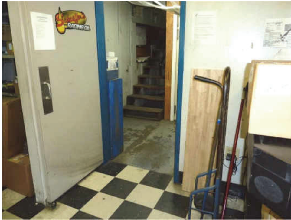
E-5. Looking southwest from office area in trailer rental center at 1535 Industrial Avenue into tool crib area with stairs to mezzanine storage area in background (06/22/2020).
