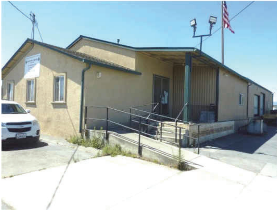
E-43. Looking southwest at Carpenter Rigging building at 1575 Industrial Avenue (06/22/2020).
