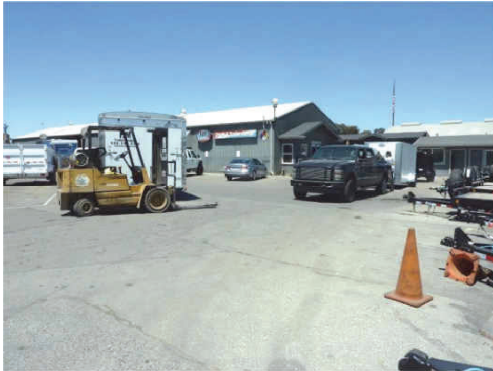
E-23. Looking northwest at trailer hook-up area outside maintenance building at 1535 Industrial Avenue with front office at right (06/22/2020).
