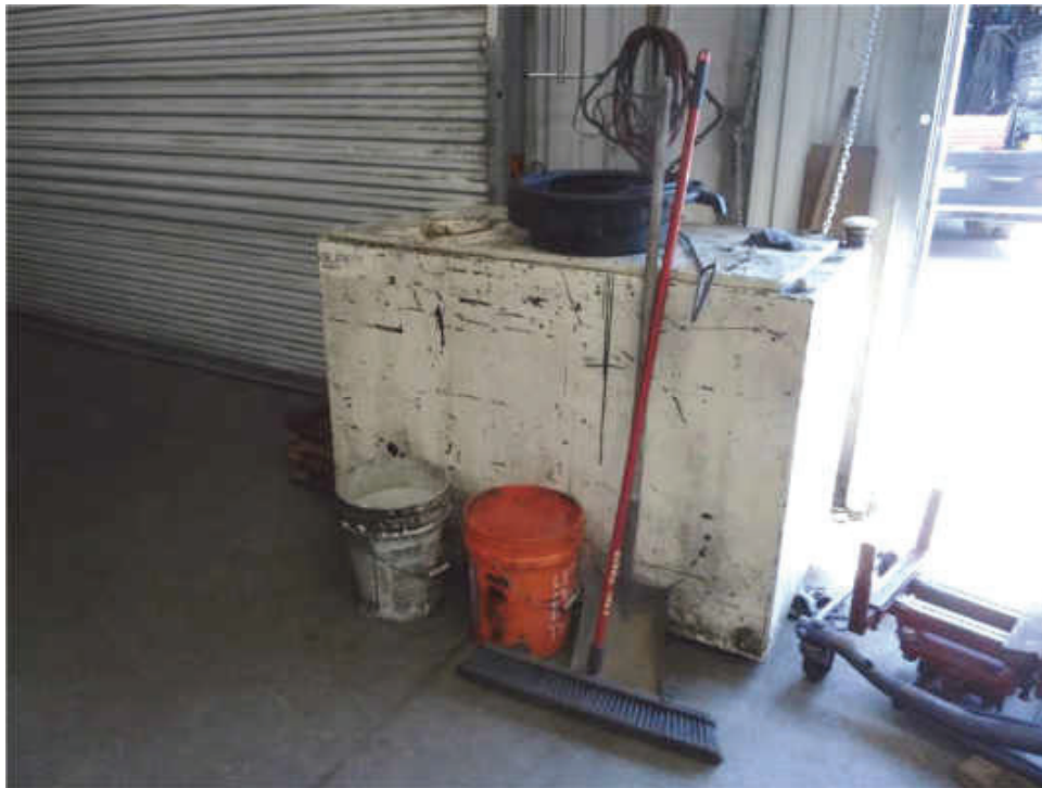
E-22. Waste oil AST inside main door into repair shop at 1535 Industrial Avenue (06/22/2020).
