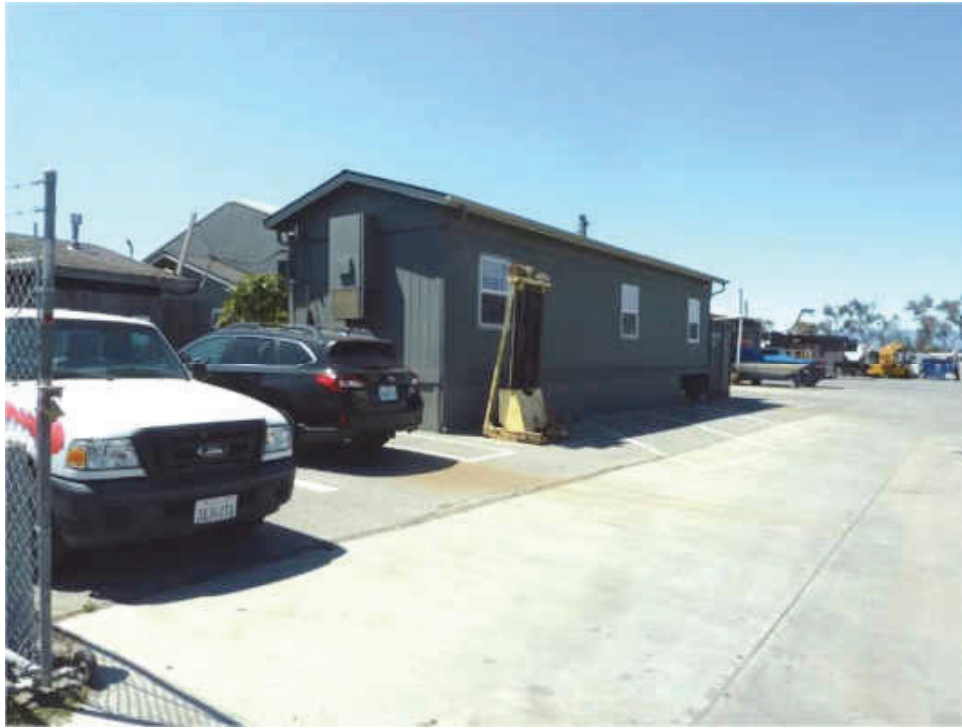
E-29. Looking southwest at rear of FJM modular office structure at 1575 Industrial Avenue, with battery storage at right and stored boat and crane in background (06/22/2020).
