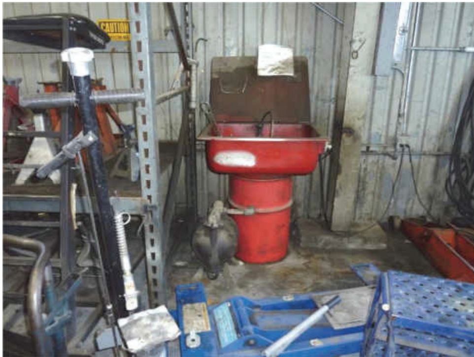
E-14. Looking northwest at tub-type parts washer in maintenance shop at 1535 Industrial Avenue (06/22/2020).
