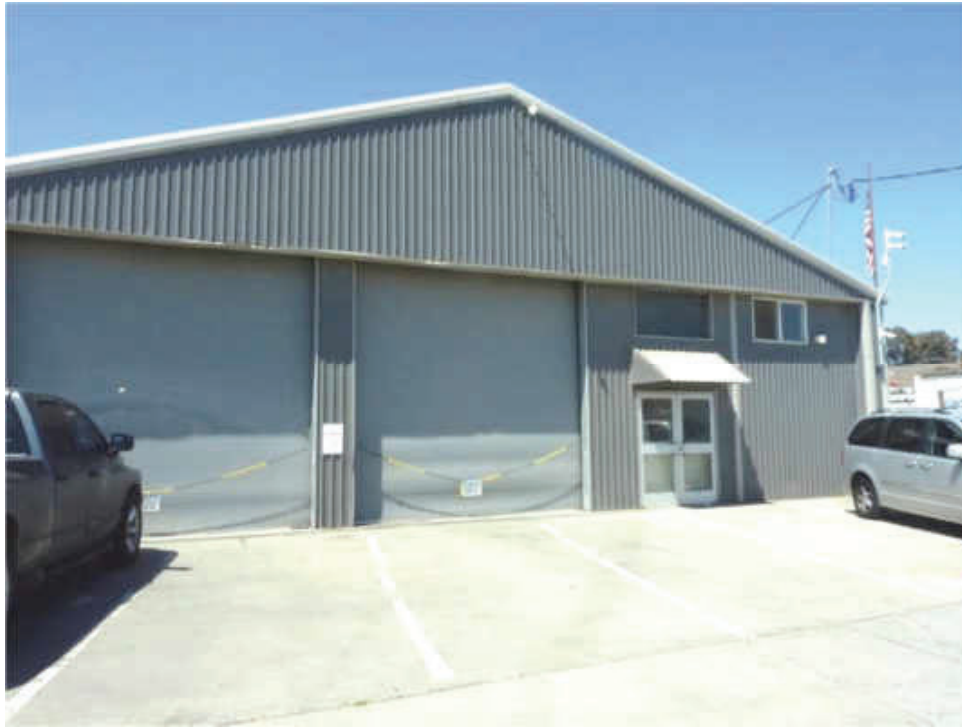
E-31. Looking southwest at truck repair shop at 1535 Industrial Avenue (06/22/2020).
