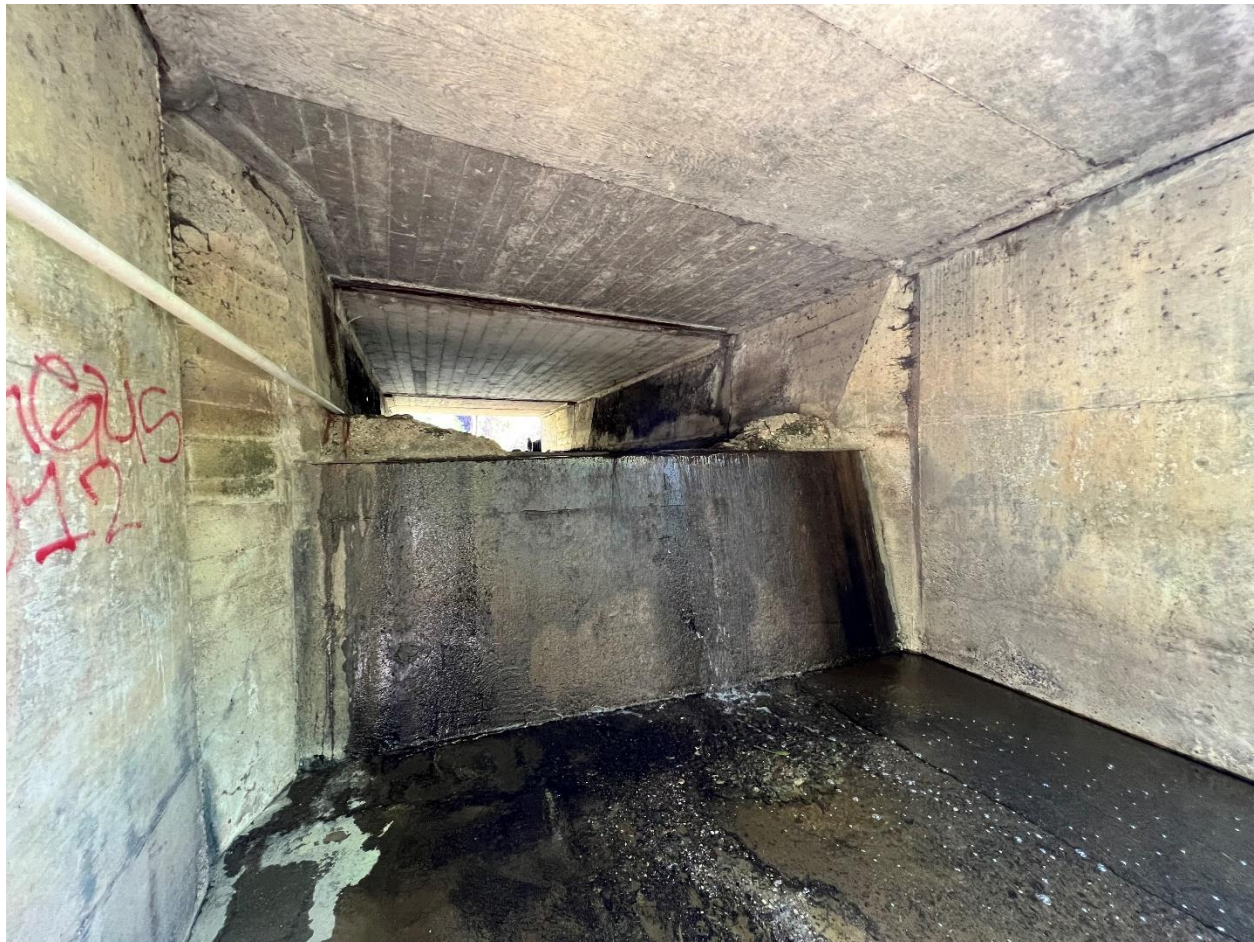
Figure 1. Location Image of Fish Passage Barrier – PM 39.2 on SR-116
