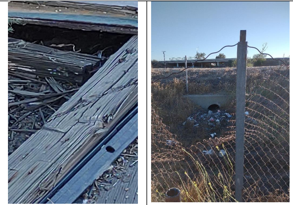
Fig 12 . 3/16/2022 (Left) Discarded pile of lumber at the west end of the project site provides potential artificial den habitat for BUOW. (Right) This culvert one of several along I-215 on the west side of the project site. This one is in the vacant lot behind Sun State Rentals.
