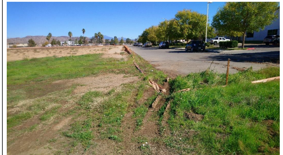
Fig 18. 11/28/2021 Looking east from the end of Exceed Road. Water sheets from the road onto the site instead of entering the storm drain at the end of the road.
