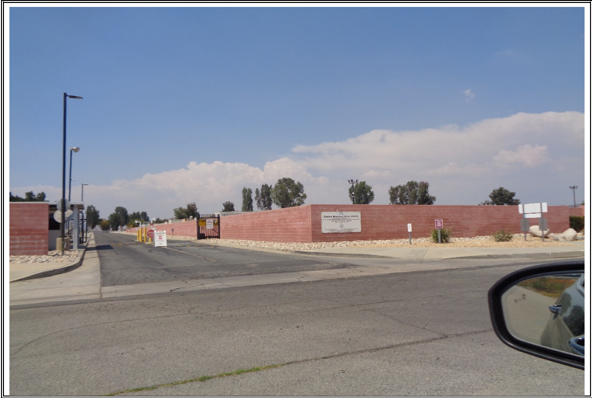
Photograph Number 20: Eastern Valley Municipal Water District to the north.
