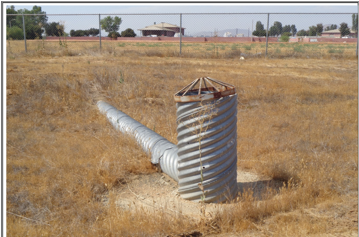
Photograph Number 10: View of catch basin located in the middle of the property.
