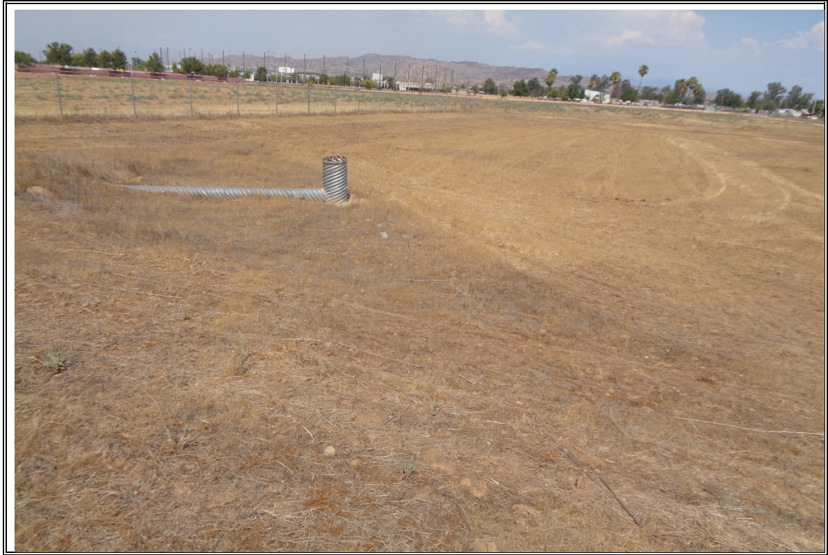
Photograph Number 11: View of catch basin located in the middle of the property.
