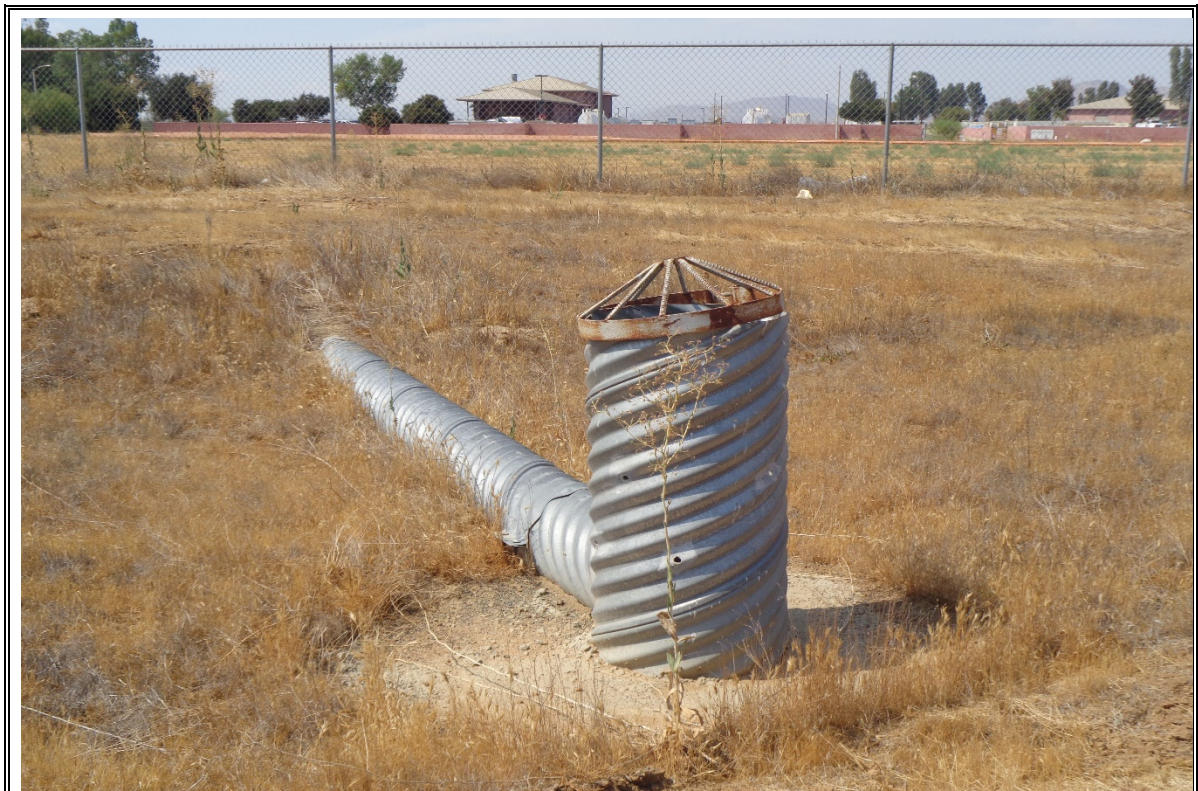
Photograph Number 12: View of drainpipe associated with catch basin running northwest.
