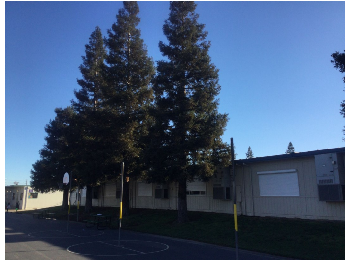
Photo 4. View of California redwoods adjacent to a building, looking northeast. Photo taken November 10, 2022.
