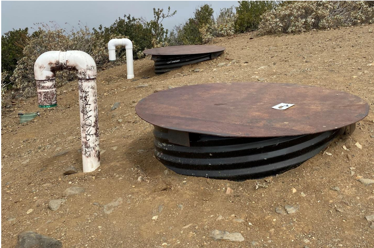
Figure 5 Modern water conveyance systems, view to the Northwest
