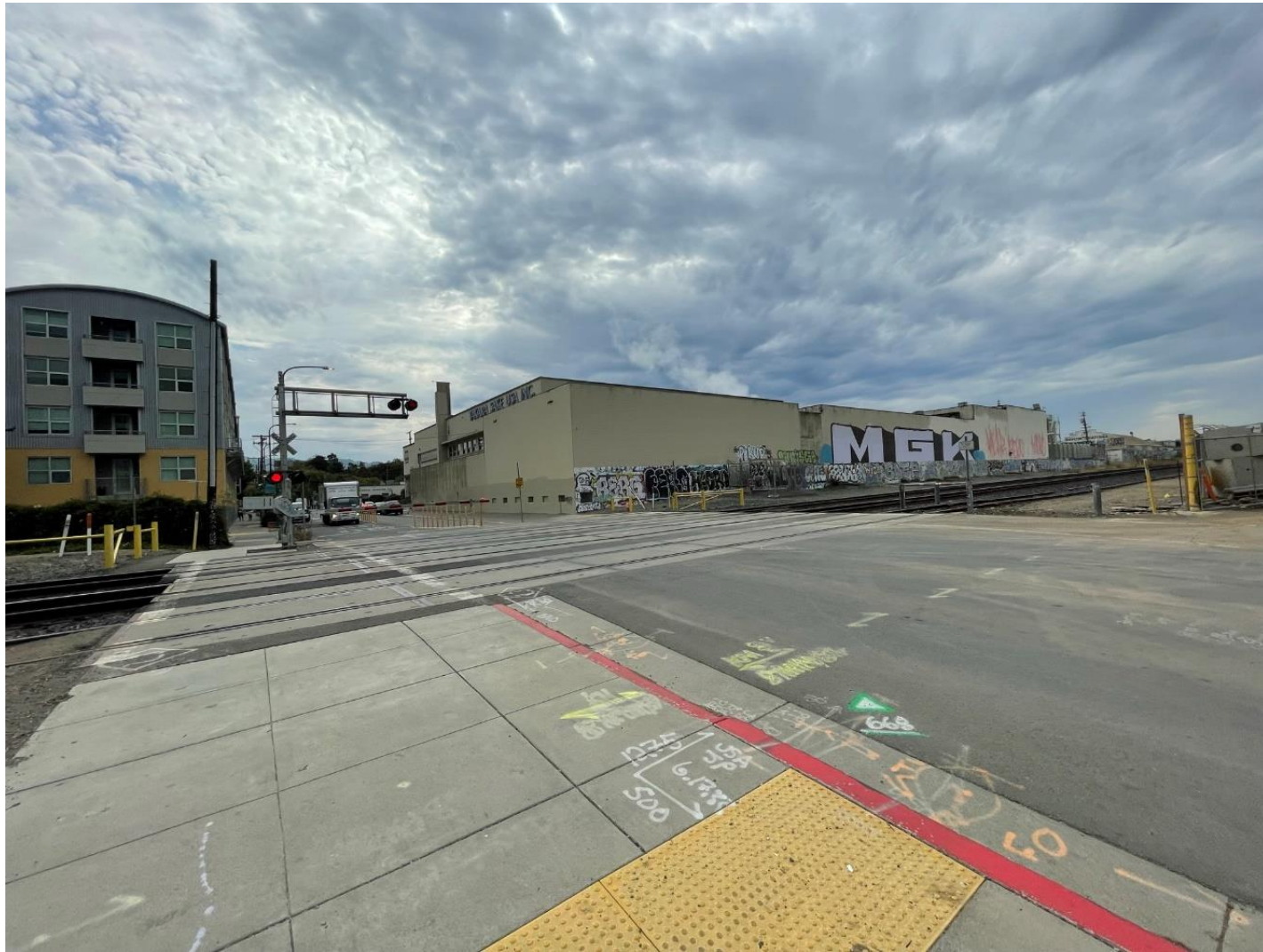
Figure 3 Addison Street Crossing - Existing Conditions
