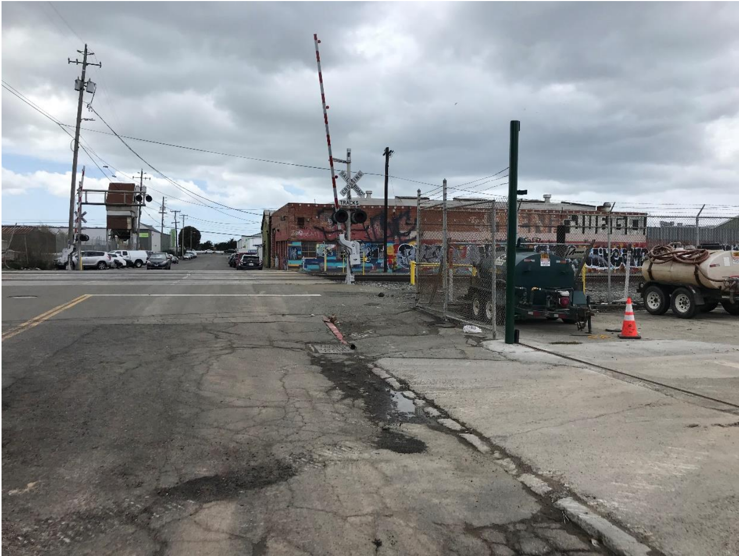
Figure 2 Cedar Street Crossing - Existing Conditions
