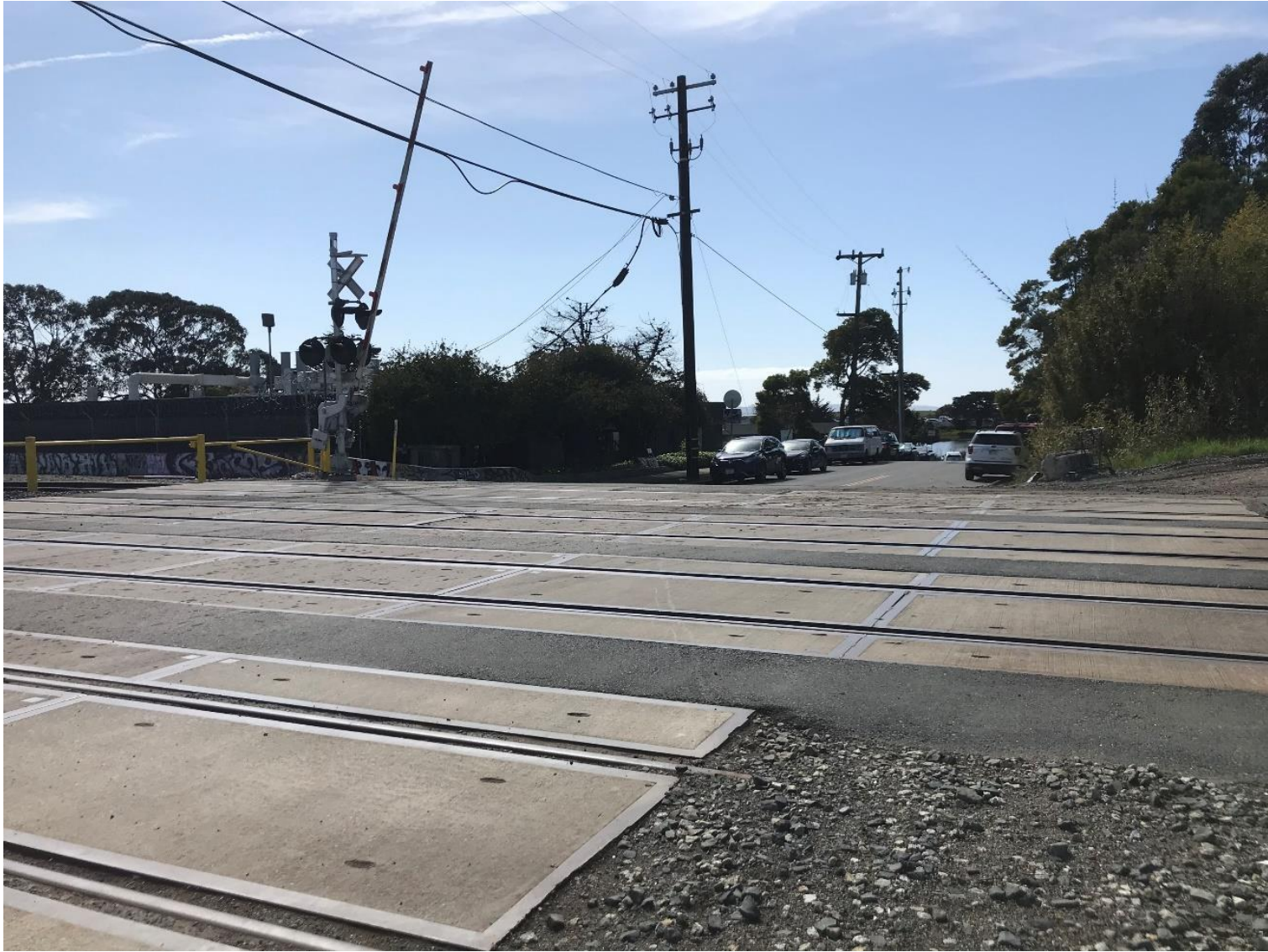
Figure 4 Bancroft Way Crossing - Existing Condition
