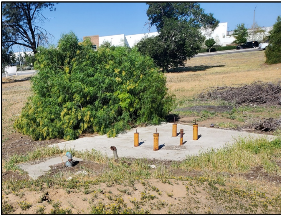
Plate 4: Overview of Feature 2, concrete slab with metal posts, facing west.
