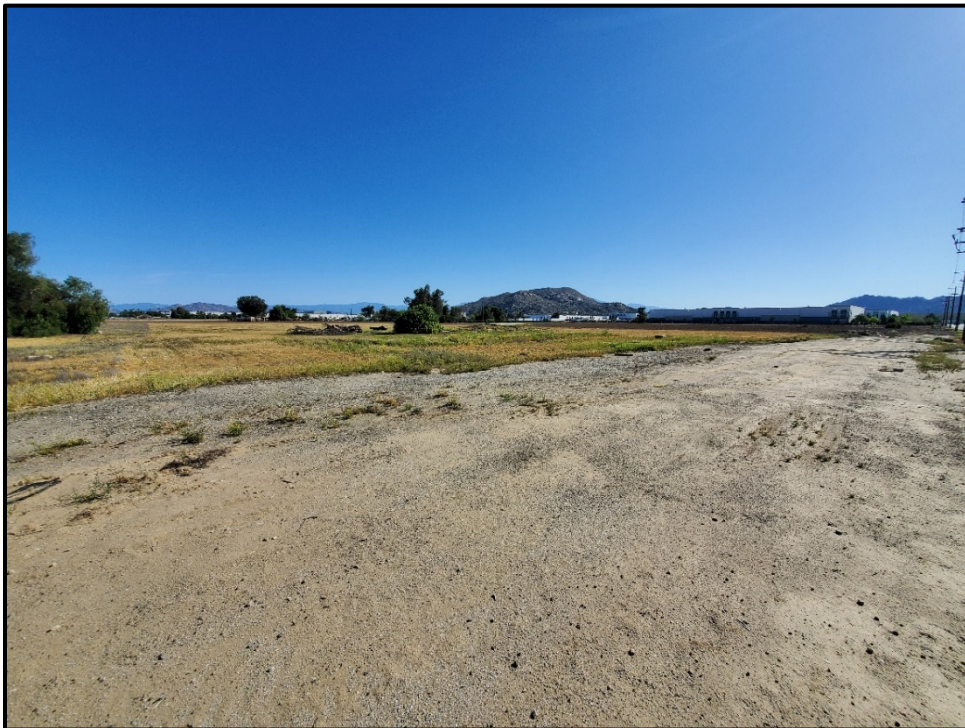
Plate 2: Overview of the Perris Truck Terminal Project from the southwest corner, facing northeast. Site RIV-8312 can be seen in the center of the photograph.
