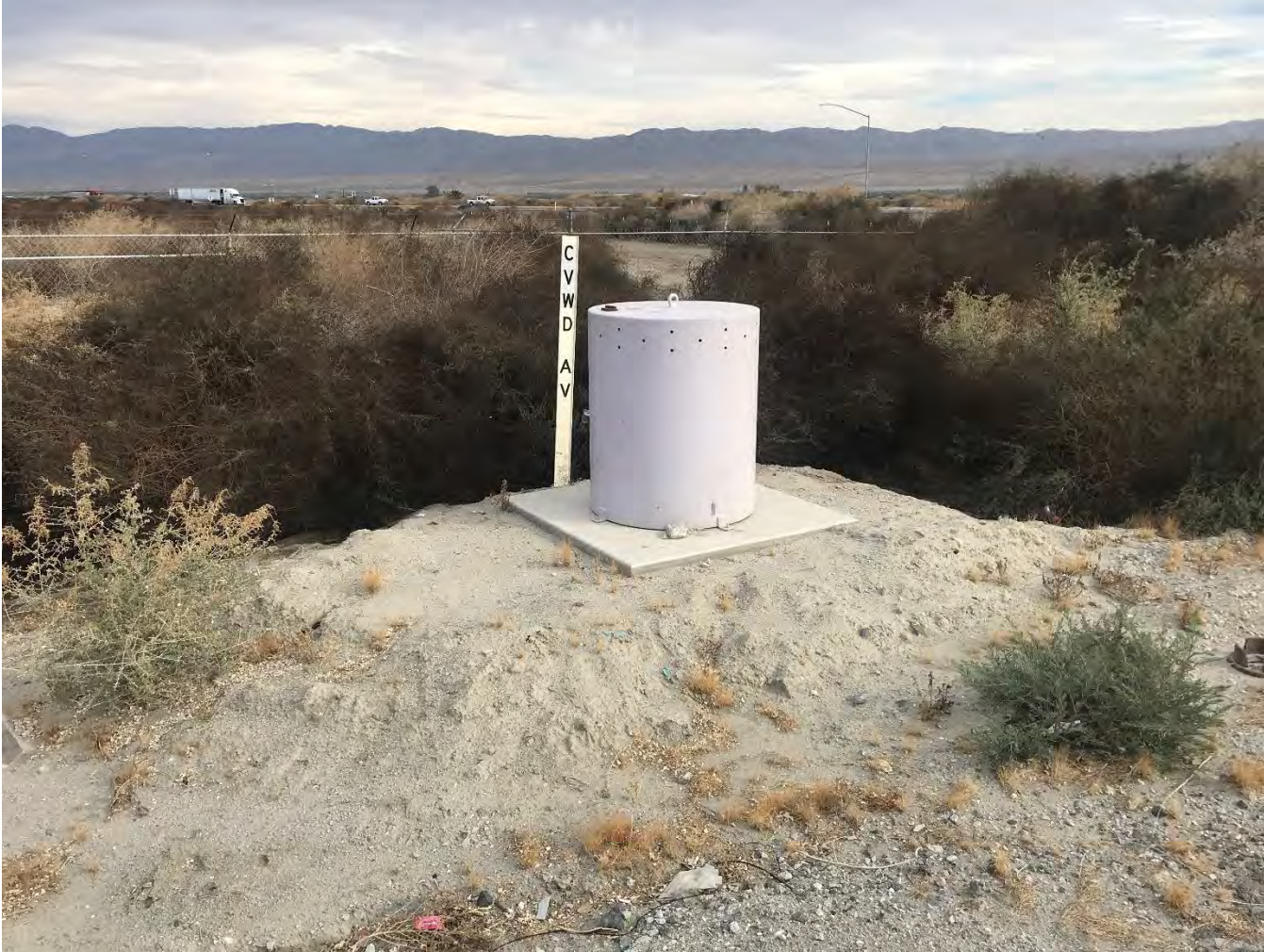
CVWD water well located along the Whitewater River channel, west of the TP, along Airport Blvd.
