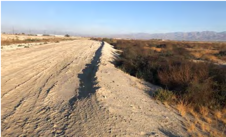
Photograph 8. Facing north, showing the start of the berm on the west side of the site that separates the site from the Whitewater River/ Coachella Valley Stormwater Channel
