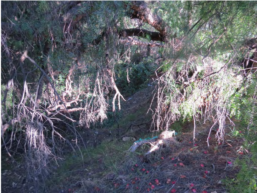
Photograph 9: View of the drainage feature on the south side of Palos Verdes Drive North.
