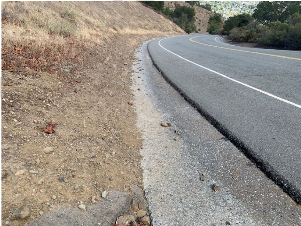
Appendix C-10. Concrete roadside ditch along Santos Ranch Road, located off the study area, looking downstream (north).
