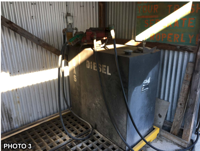
SOUTHERN PARCEL - ABOVE GROUND DIESEL STORAGE AND REFUELING TANK
