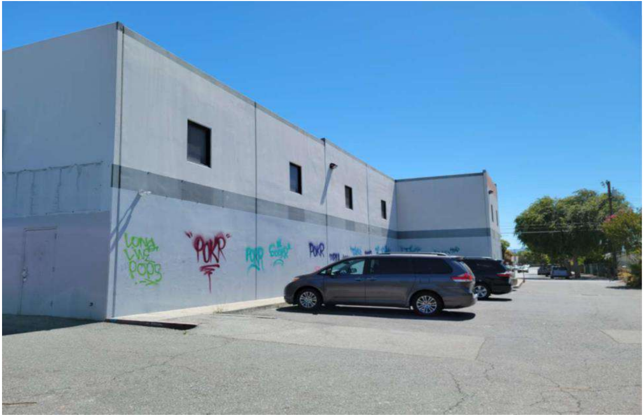
Photo 4: North side of the existing retail commercial building.
