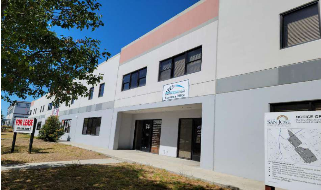
Photo 1: Existing two-story retail commercial building located at 70-80 N. 27th Street. This building would be demolished as part of the project.
