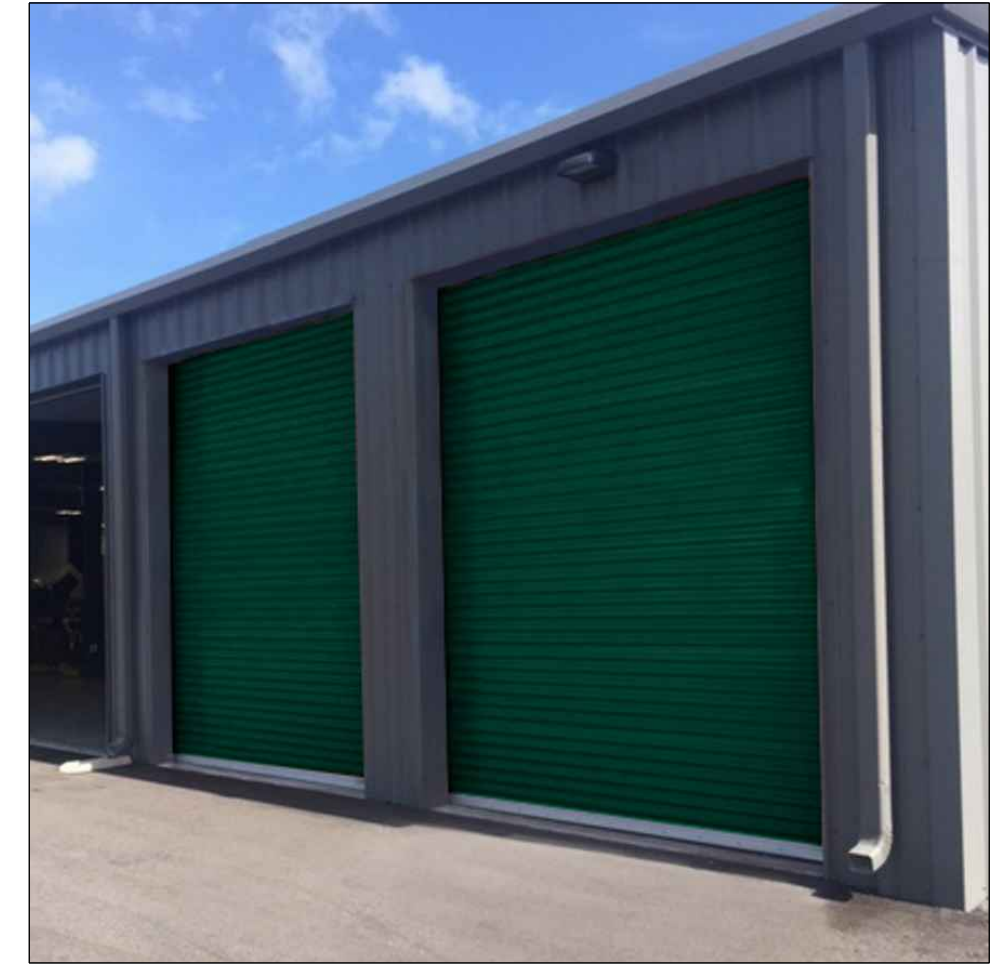
FAUX UNITS/ EXTERIOR ROLL-UP DOORS MANUFACTURE: JANUS INTERNATIONAL COLOR: LG (FOREST) GREEN (OR APPROVED EQ.) C4
