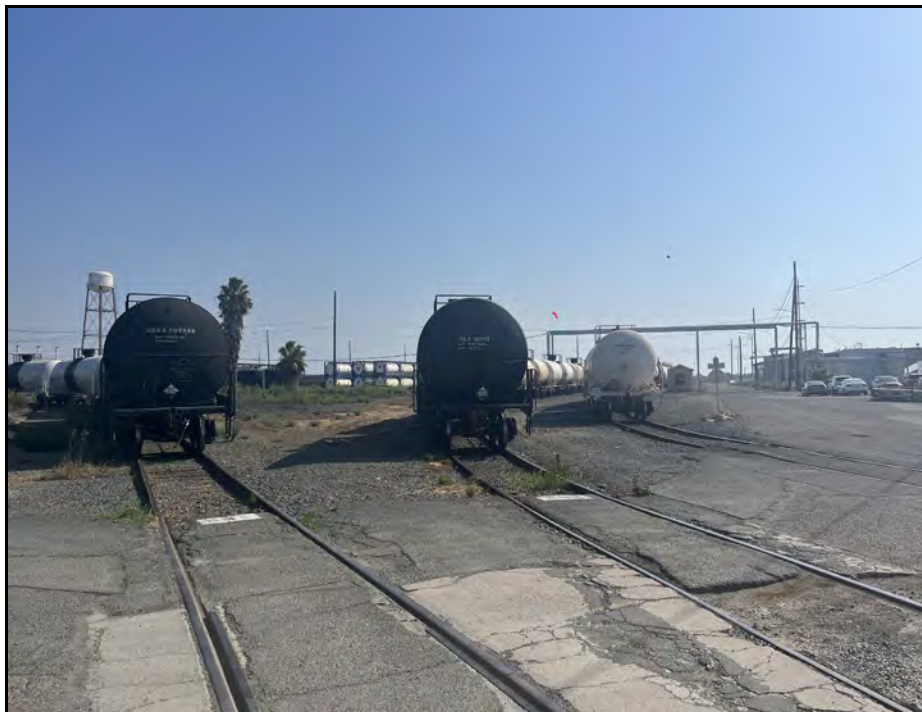
Figure 8. Overview of resource P-07-000806/CA-CCO-372 (railway spur); view to the south.
