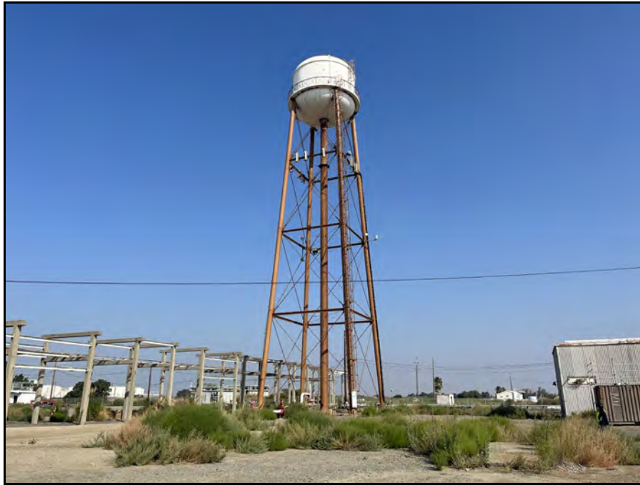
Figure 7. Overview of east section of Project and resource REJ-092223-STR-01. View to the northwest.
