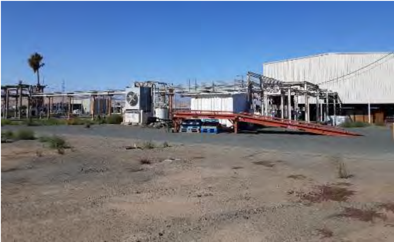
Photo 4: Site overview – looking southwest (Photo Date 8/25/2023)
