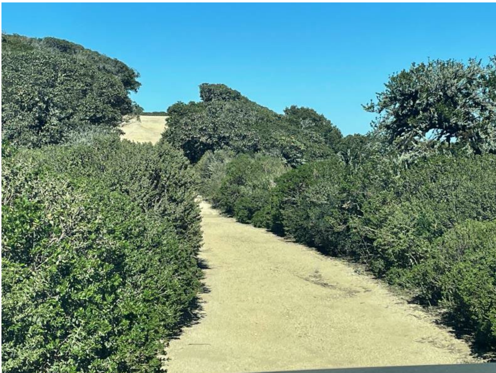
Photo B-2. Coyote brush scrub encroaching into the roadway (2/8/2022)
