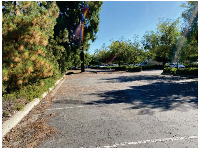
Photo 6: View from southwestern corner looking north.
