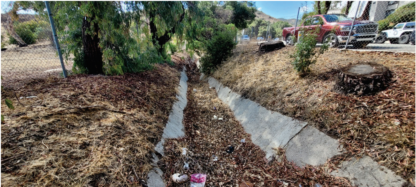
Photo 8: Typical view looking south at Drainage 5. Photo Date September 15, 2022
