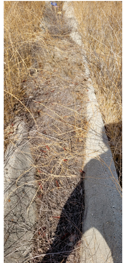
Photo 6: Typical view looking west at Drainage 4. Photo Date September 15, 2022
