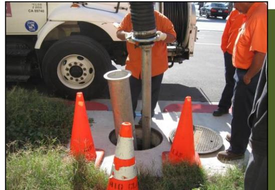
Insertion of vacuum hose into separation chamber.
