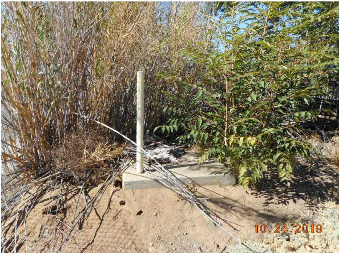
**Photo 12** - View facing west showing a concrete pad in/near the southwest corner of the subject site. Within the concrete pad (5' by 5') is a steel manhole cover, labeled "YVWD SEWER", likely an acronym standing for Yucaipa Valley Water District sewer.
